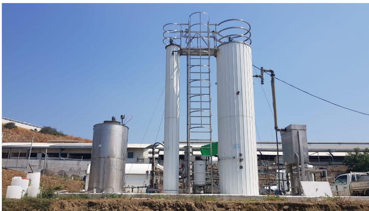
Figure 1: Struvite precipitation plant in Cyprus
