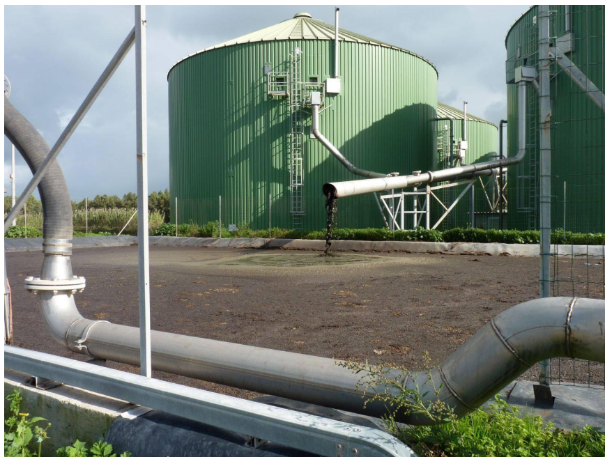
Figure 2: Bio-digestate in Arborea to be treated in the Struvite precipitation plant
