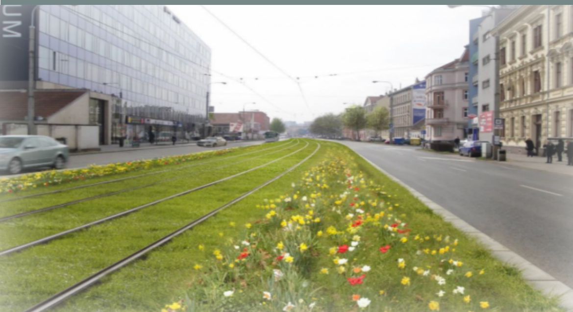
Figure 7: Visualization of reconstruction of tram lines Nové sady in Brno, where the “green belt” - meadow lawn with flowers - will be built for less noise and dust. Source:
