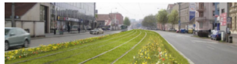
Figure 7: Visualization of reconstruction of tram lines Nové sady in Brno, where the “green belt” - meadow lawn with flowers - will be built for less noise and dust. (Source: www.dpmb.cz 2020)
