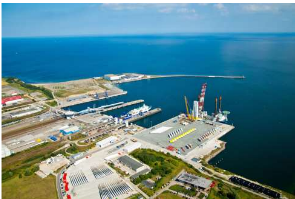
Figure 83. Installation of OWF „EnBW Baltic 2”, Mukran Port.
