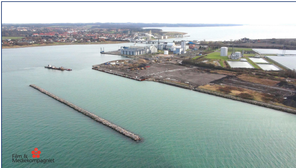
Figure 64. Initial expansion stages of Vordingborg Port using recycled materials
