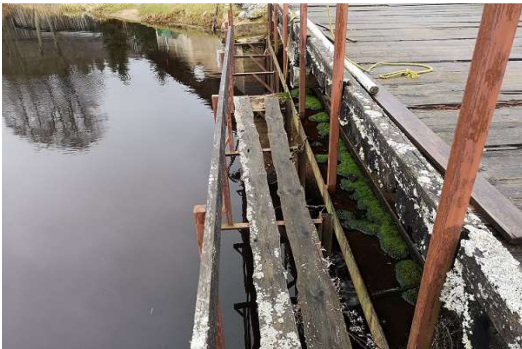
Photo 19. Removing stoplogs from the excess water outlet is a life threatening operation, especially in the winter, when logs are frozen or snowy and the stoplogs are stuck. By the way, this is usual for many of the Estonian dams – if there is a fast need to remove stoplogs, then often it is not possible (R. Järvekülg, 08.12.2019).
