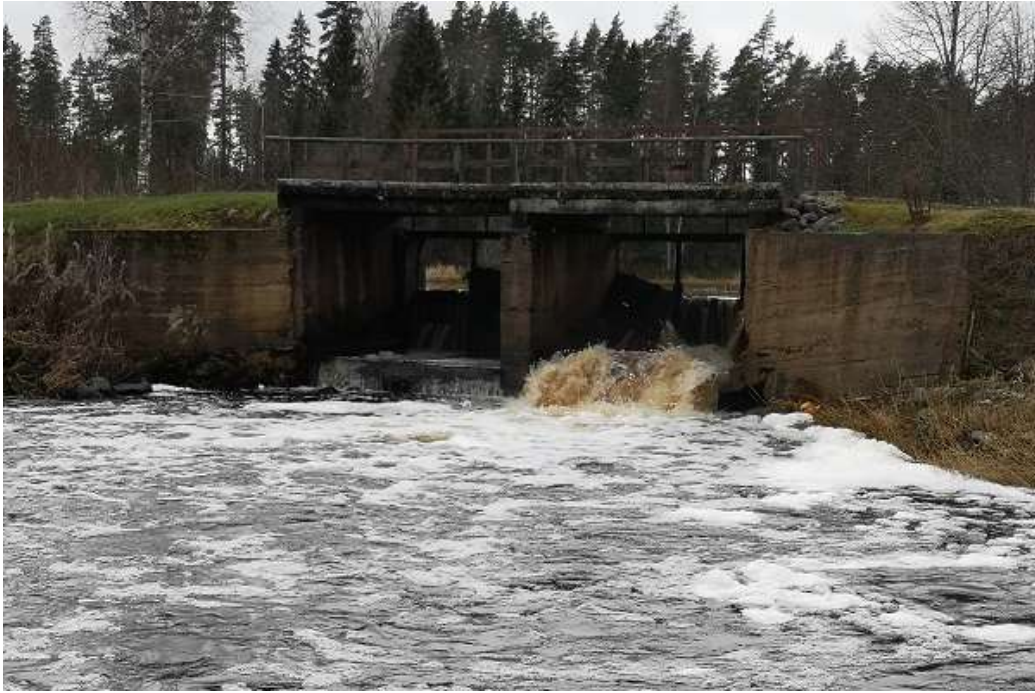
Photo 18. Dzirnavas dam's water level is raised by ca 2,1 meters. During high water some of the stoplogs are removed and therefore the expansion level is lower. On the day of the observation only the left excess water outlet was partly open which is achieved by removal of the stoplogs. Dam's owner is concerned with the unexpected openings of the Holdre dam, after which there is a risk of flooding in the Dzirnavas dam (R. Järvekülg, 08.12.2019).
