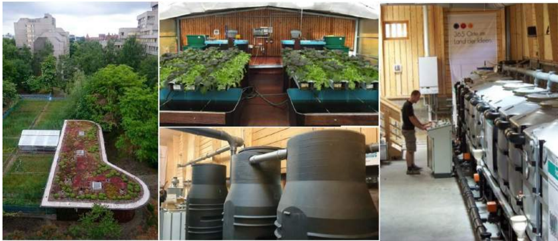
Fig.1. Photos of the ROOF WATER-Farm system (from left to right and top down: test site, greenhouse, blackwater treatment plant and grey water treatment plant [biological fluidized bed processes])
