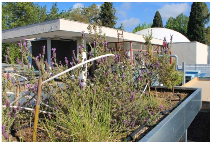
Fig. 3. Test bed with vascular plants and mosses at the rooftop of the Herbarium building at Instituto Superior de Agronomia, University of Lisbon.
