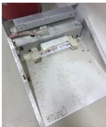
Fig. 7 – Corridor projector: old systems with 250 W lamp
