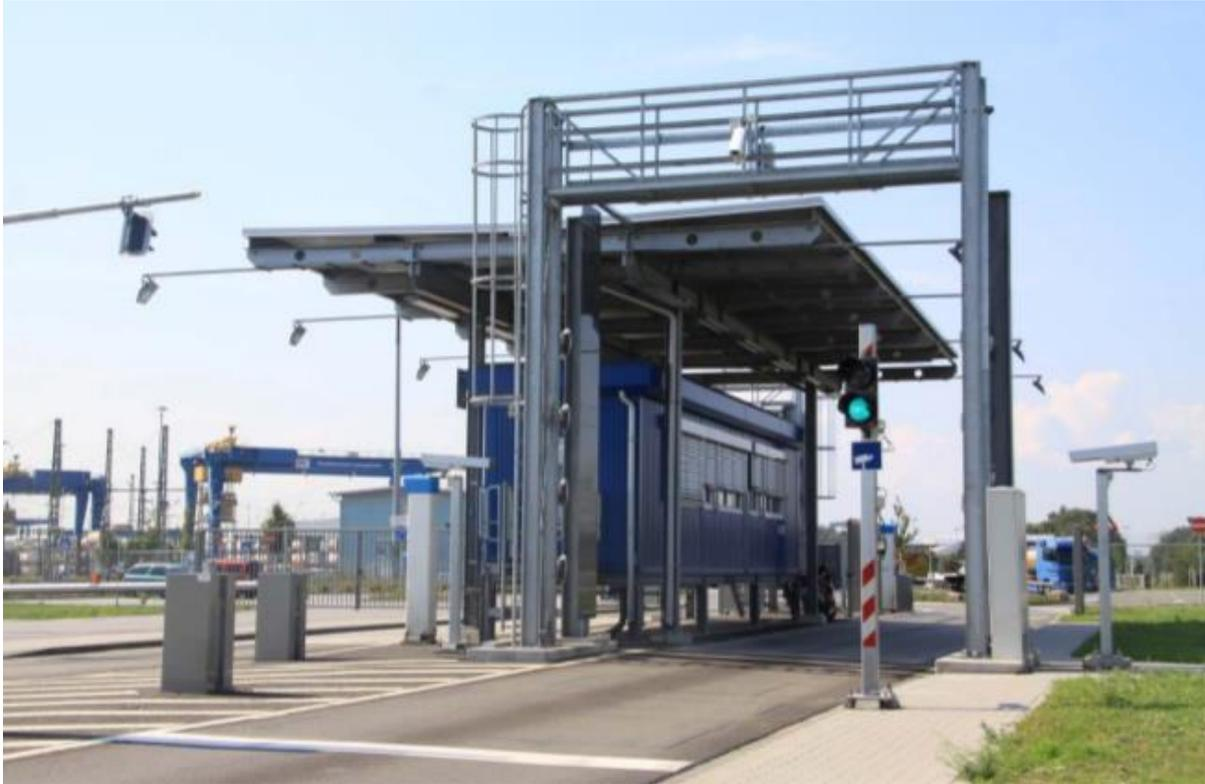
15. Figure - OCR gate automation at KTL Kombi-Terminal Ludwigshafen GmbH.
