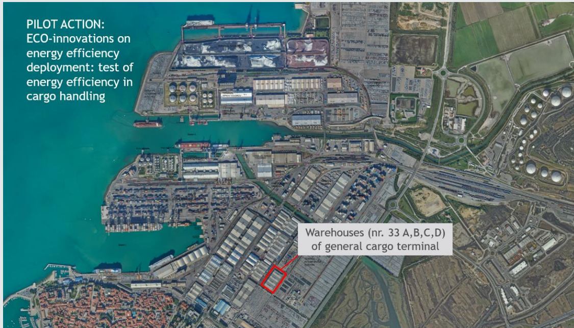
Picture 2: Location of the Pilot action (warehouse nr.33 of the General cargo terminal)
