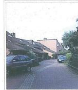
A purpose designed woonerf in east Utrecht
