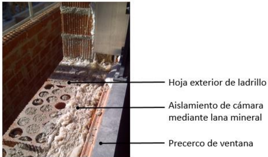
Image 22. Intervention in contour of windows with facades with air chamber.
