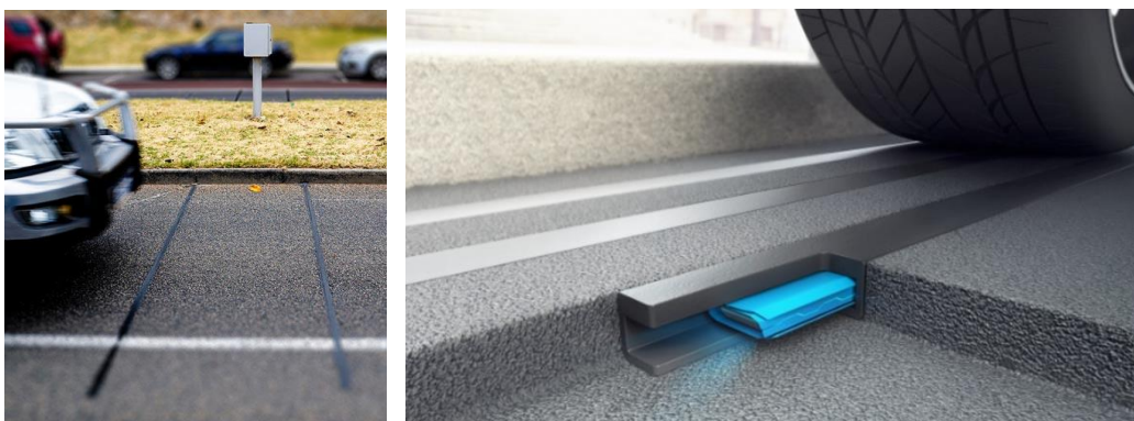
Figure 13: Piezoelectric detector, source: (9) (10)
