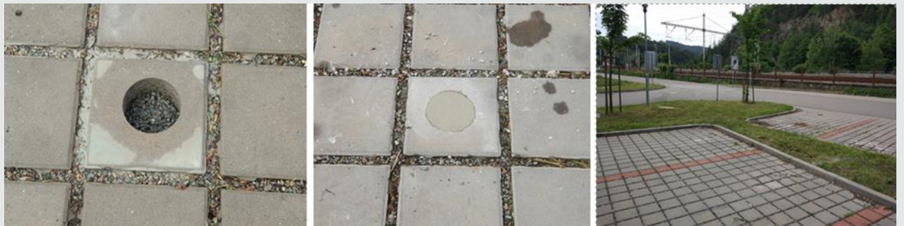
Fig 02: Installation of sensors at parking spot
