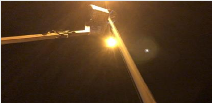
Fig -01-02 - Cameras installation in September 2018 at night
