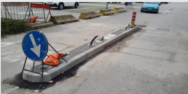
Fig 01-02-03 - Preparatory works for installation of inductive loops and barriers
