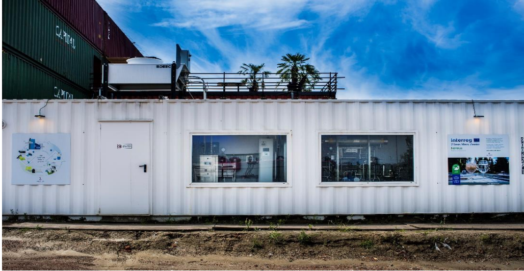
Figure 2 - Water-link's pilot plant
