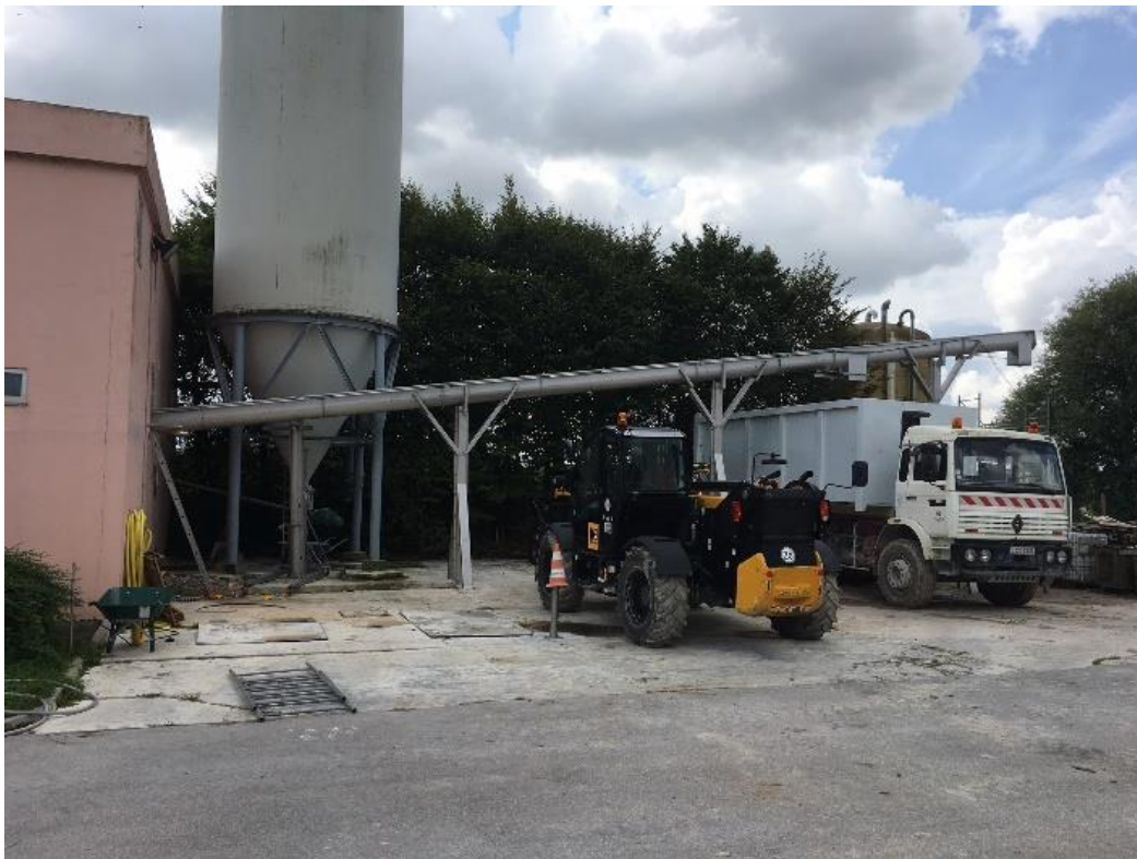
Figure 3 - Saint-Omer wastewater treatment plant
