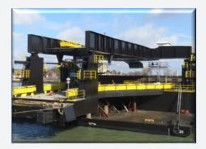
Portsmouth port installed a **new linkspan** which takes **more weight** and **operates more quickly**. This allows the ship to make her channel crossing slower allowing for **fuel savings** and **reduced carbon production**. This will result in far **fewer emissions**.
