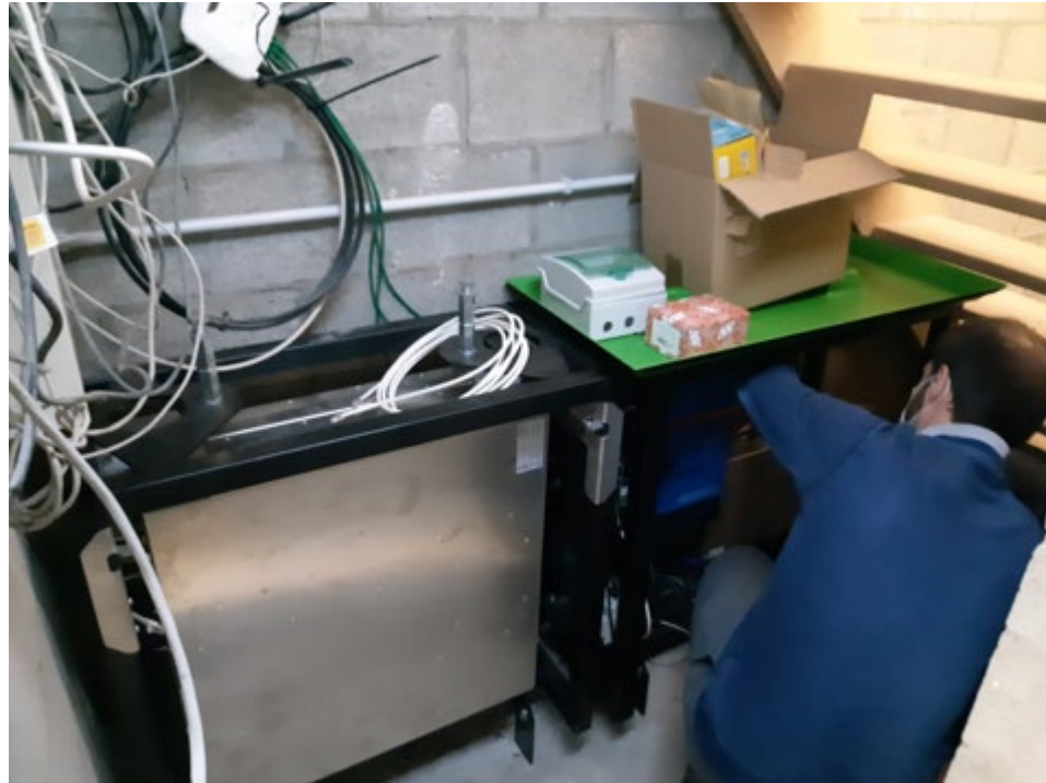
This picture shows the battery system being installed.
