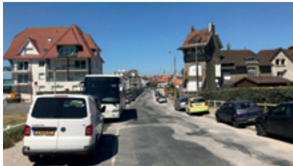
Before work started
