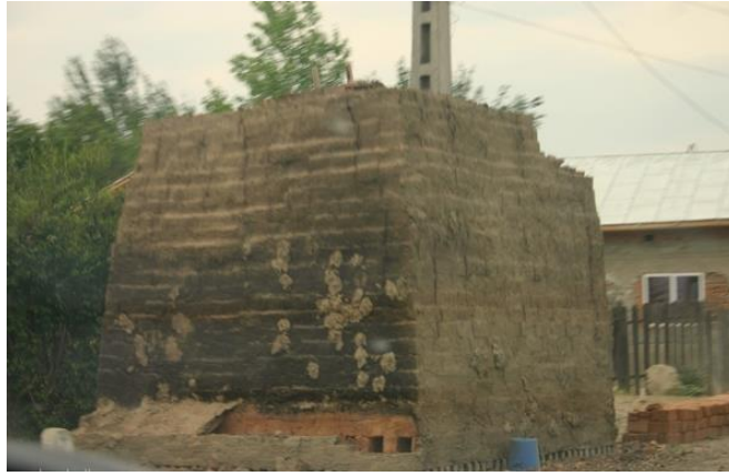
Furnace for brick
