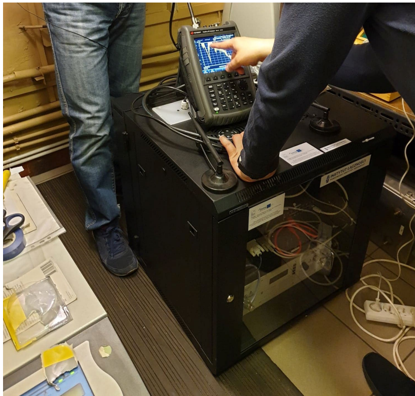
Figure 2-17: Installation of the transmitting station in Gdynia
