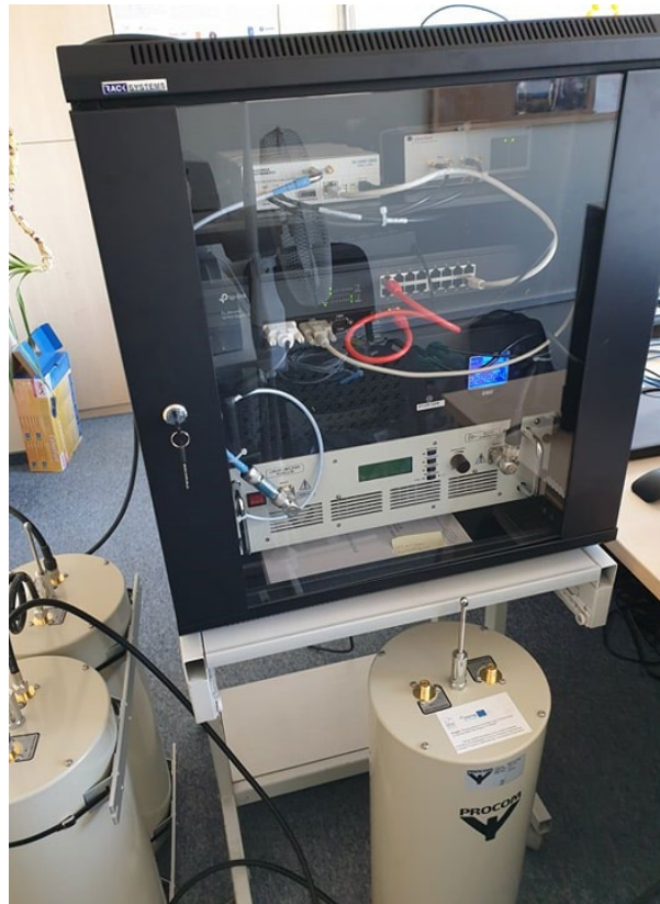
Figure 2-13: Front of the transmitting station
