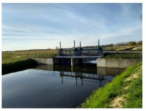
Photos. Damming water by hydrotechnical facilities, Moszczenica River, Bedlno Commune; the water is redirected to irrigation ditches
