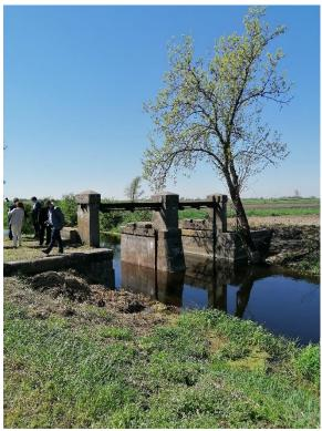
PHOTOS: The non-functioning weir causes drainage of water from adjacent drainage systems. Note the water level in the riverbed during the dry (2019) and wet (2021) years.
