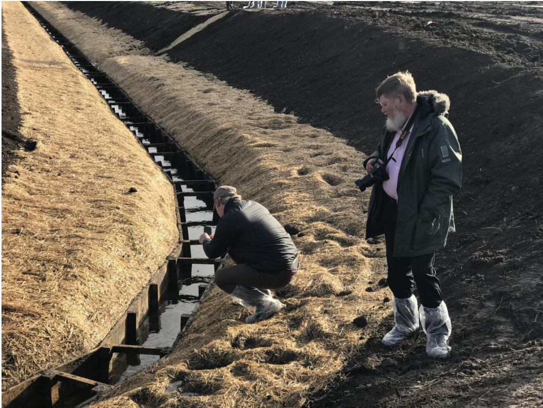
Figure 3. The Sodite stream after renovation (14.11.2017)
