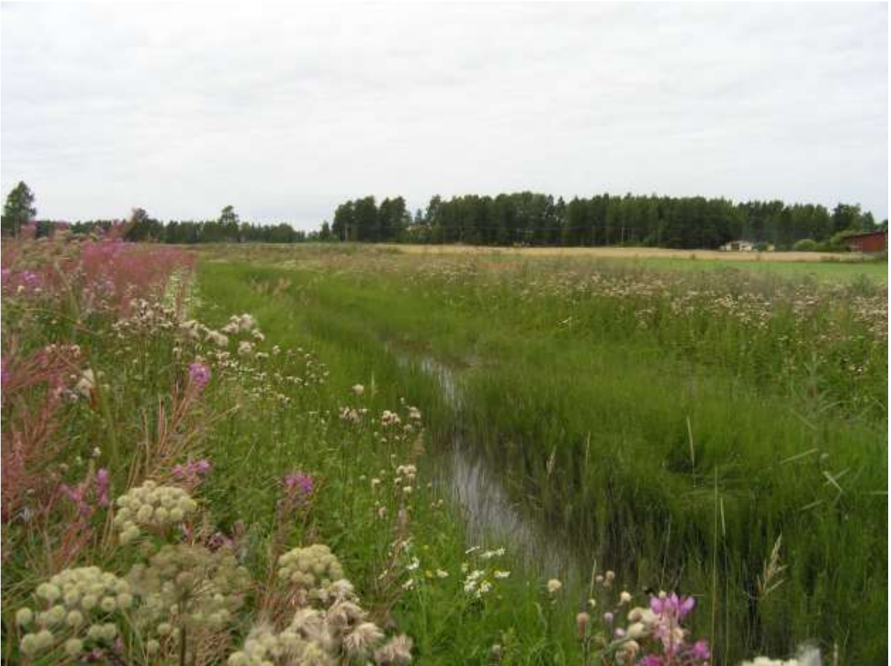
A two-stage ditch, with both flood plain on both sides. Photo Mikko Ortamala
