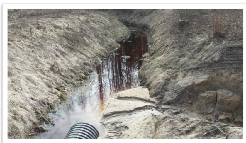
Photo 2. A ditch in Latvia which should not have been cleaned because of the highly erodible soil causing high sediment load to downstream water bodies. Photo Zane Libieté.
