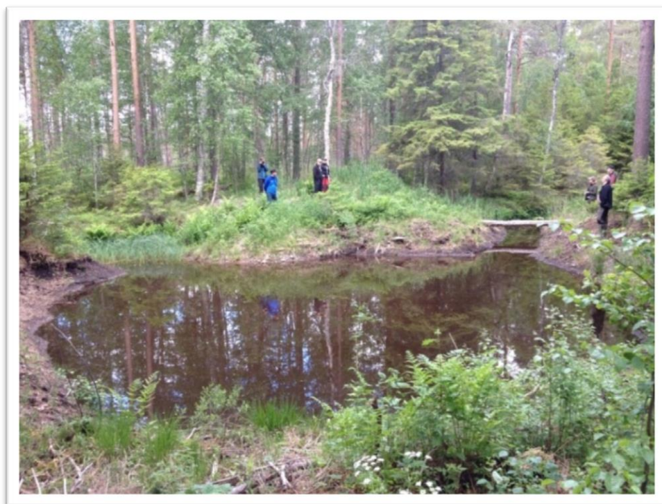
Figure 5. Top: Schematic diagrams of a sedimentation pond with recommended dimensions for retention of suspended solids. The outflow ditch is not cleaned. Cross-section A-A1 of the pond is illustrated on the right (Drawing Ilze Paulina). Bottom: The photo shows a sedimentation pond in Sweden (Photo Ulf Sikström).
