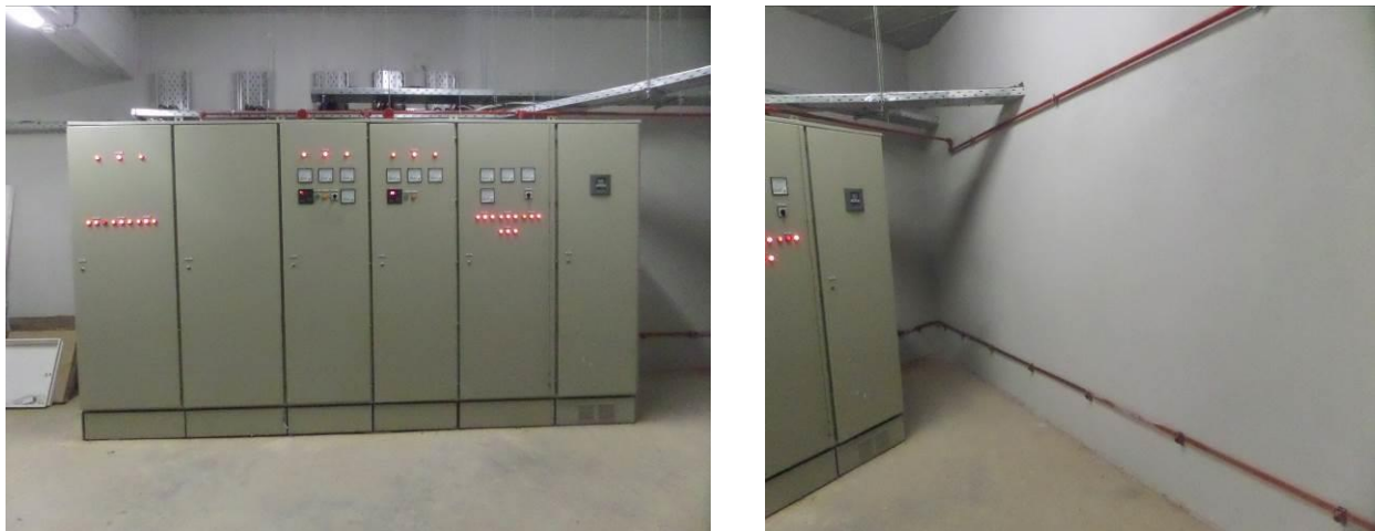
Figure 7: Inverters and storage asset installation room
