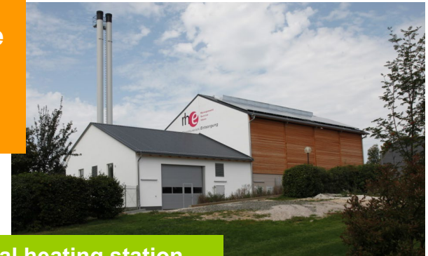
Central heating station
