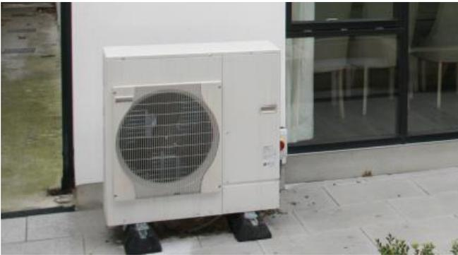
Heat pumps are machines that extract heat from one place, upgrade it to a higher temperature and move it to another place. Heat pumps work by circulating refrigerant liquids between two heat exchangers with a compressor pump.
