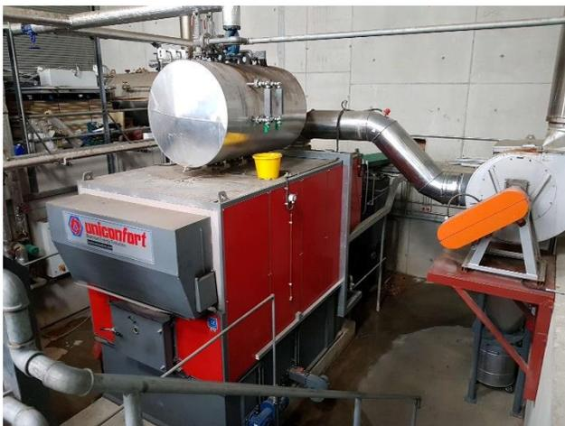
The appliance will determine the wood chip used (quality, size, moisture content). Output is usually (much) larger than 30 kW. The wood chip market is currently developing rapidly. Domestic-scale wood chip heating systems require a chip moisture content of approx. 25% by preference. Larger systems can handle moisture levels of 35 to 45%.
