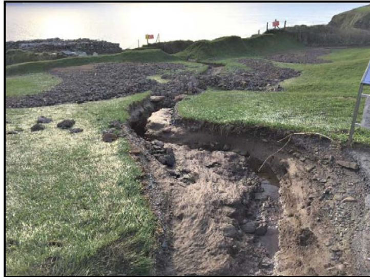
Figure 6. Flood damage at the site in 2017, with scoured areas and deposited heavy gravels (© NMS)
