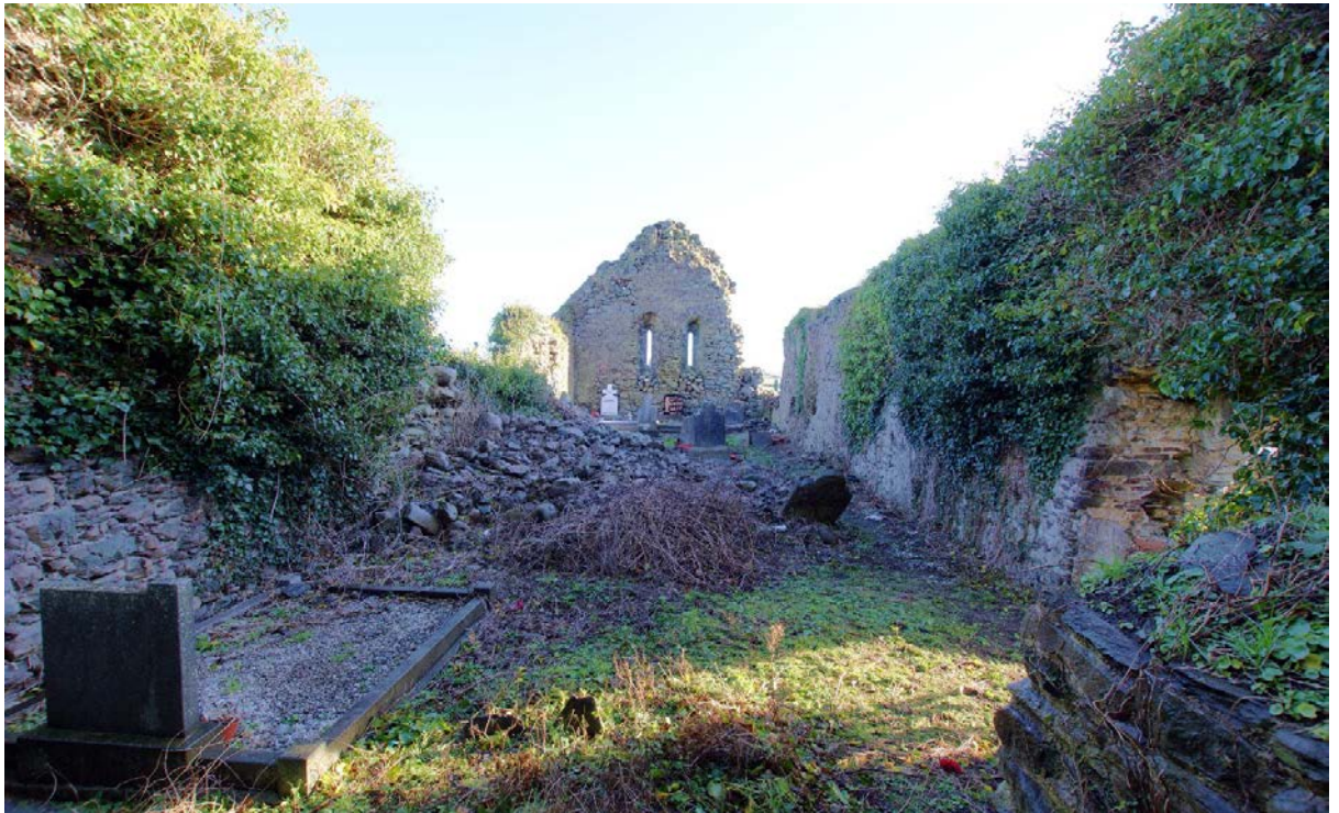
Figure 5: Kilbonane Church which was structurally intact in 2009. The major collapses at this site occurred after an extended period of freezing weather in 2010 and heavy rainfall over the Autumn of 2012
