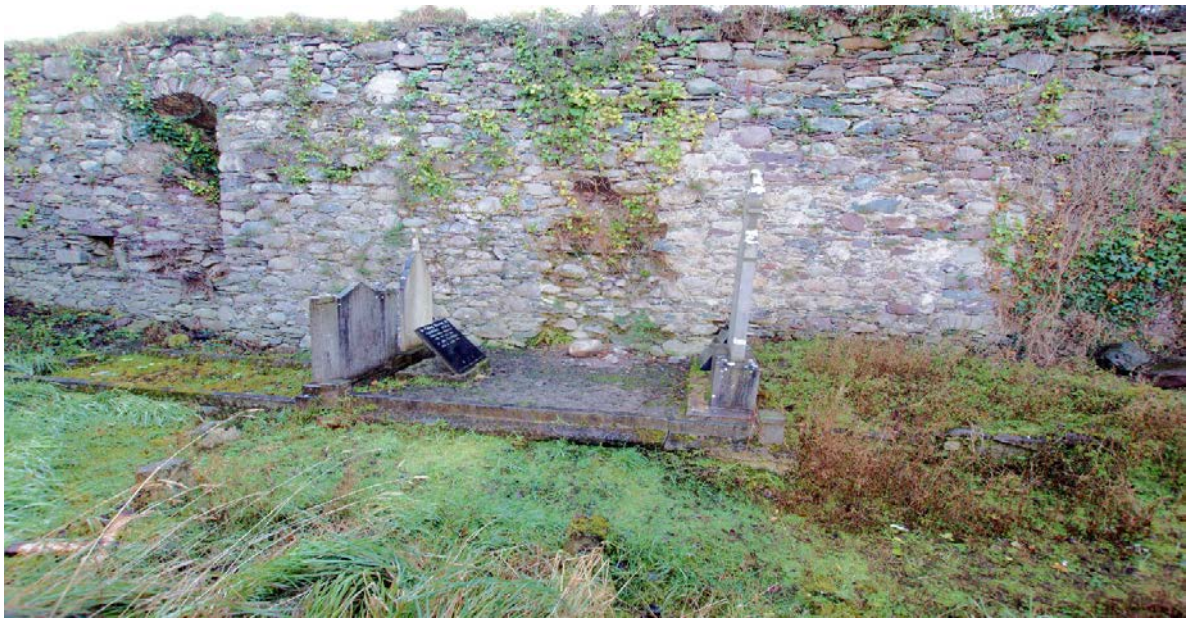
Figure 5: Grave surround cut partly under side wall at Churchtown causing slumping and cracking of the wall. Note recently fallen stone from the wall face
