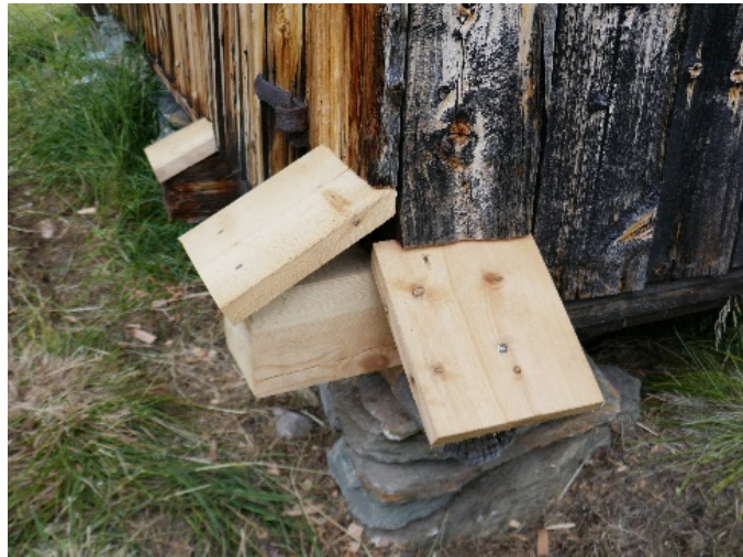
Figure 3 Solution to avoid rot damage.
