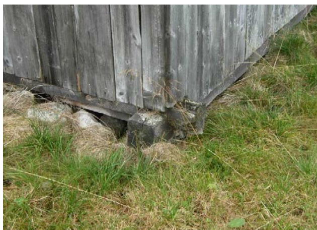
Figure 2 Damage caused by brown-rot.
