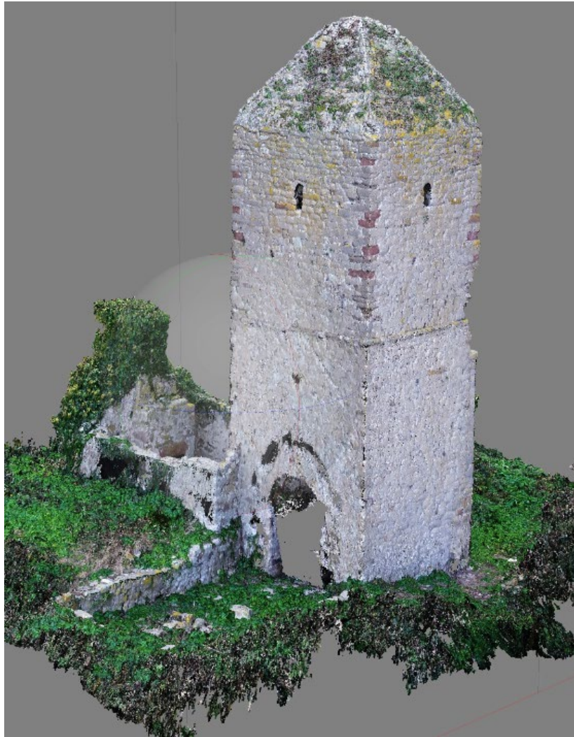
Figure 18 Puffin Island. Photogrammetric model of the twelfth century church tower seen from the north-east; dense point cloud produced using Agisoft metashape from 186 photographs flown by a UAV (Crown Copyright: CHERISH Project).
