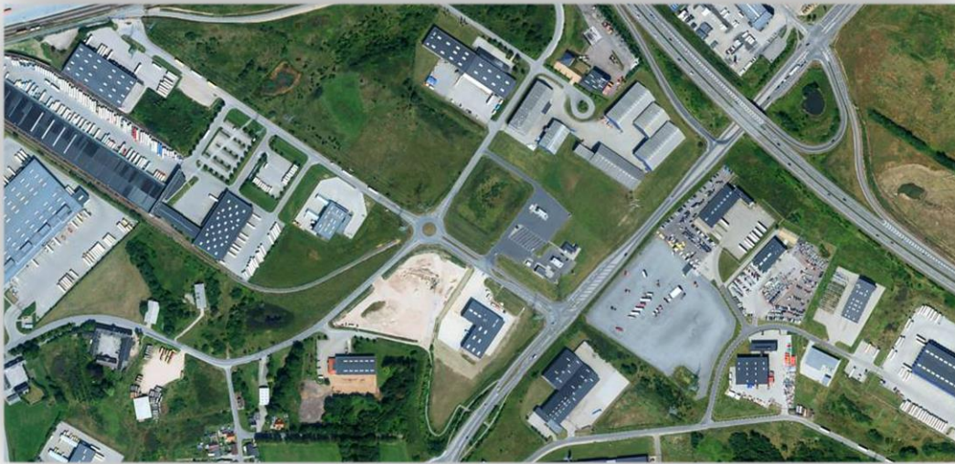
Figure 13 - Picture of fuelling area at Taulov Transport Centre with nearby gas grid
