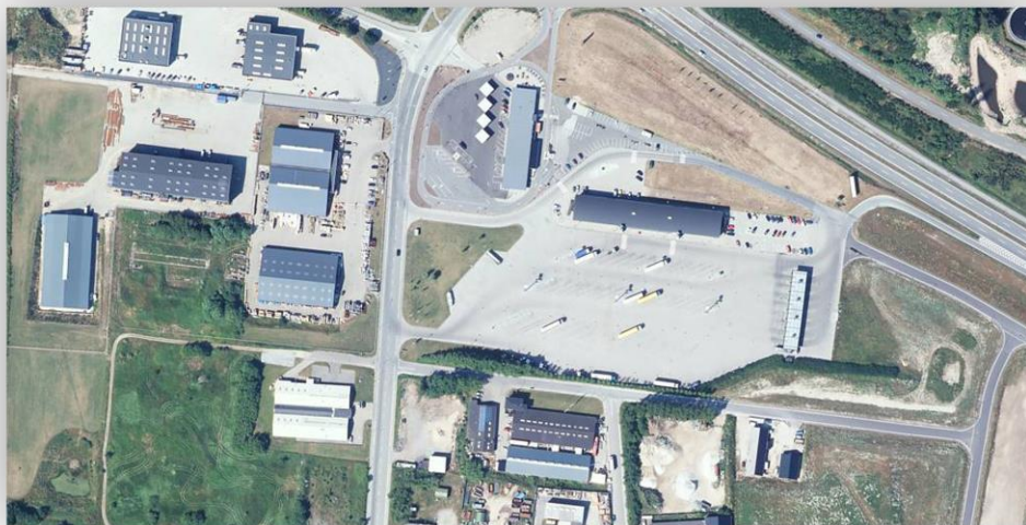
Figure 9 - Picture of fuelling area at Hirtshals Transport Centre with nearby gas grid
