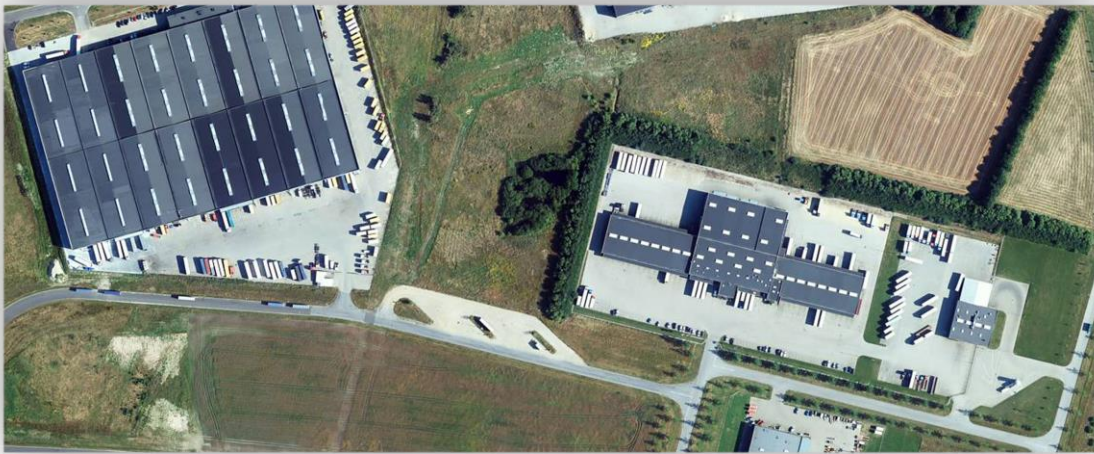
Figure 11 - Picture of fuelling area at Herning Transport & Logistics Centre with nearby gas grid
