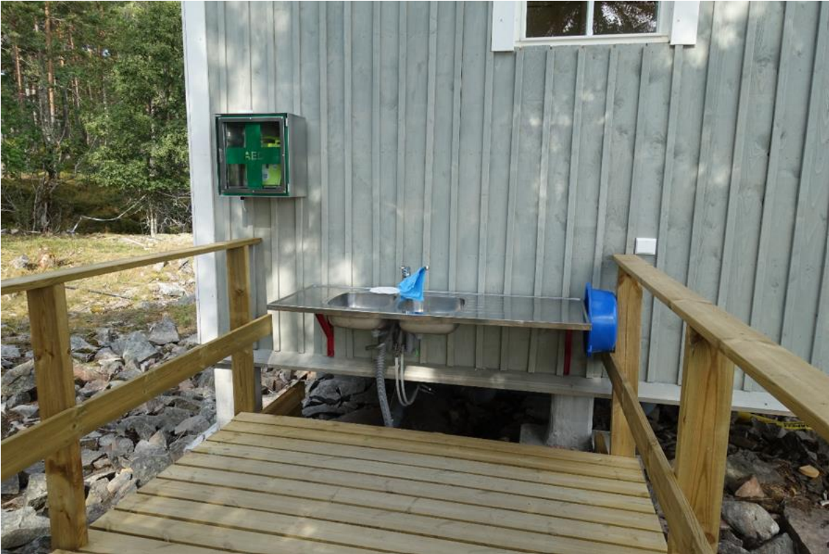
An AED defibrillator unit and a dish washing facility are installed on the outside wall of the service building. Photo: Metsähallitus / Sanna-Kaisa Juvonen.
