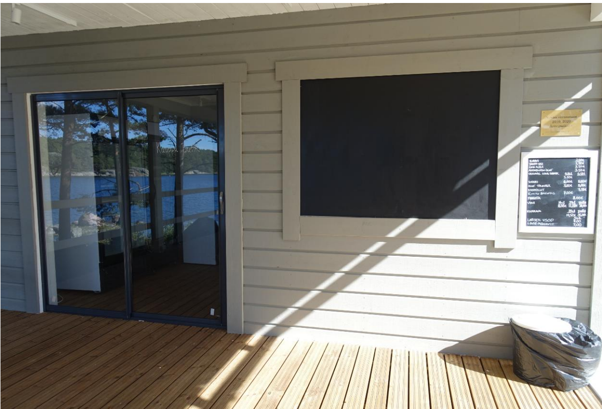
Service hatch and entrance from the terrace to the new service building. Photo: Metsähallitus / Sanna-Kaisa Juvonen.
