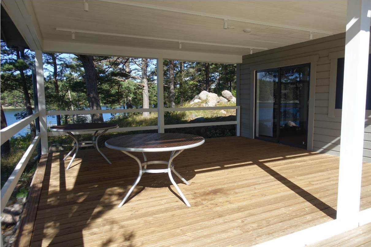
Terrace of the new service building. Photo: Metsähallitus / Sanna-Kaisa Juvonen.
