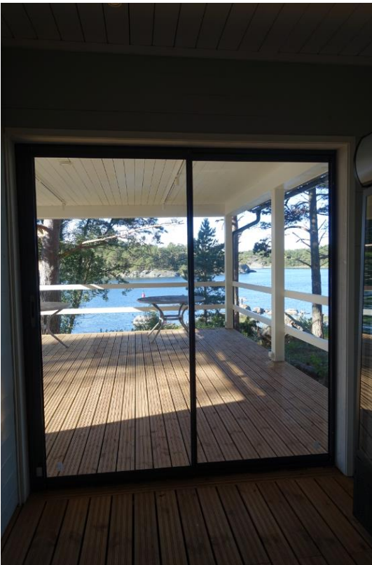
View from the inside of the service building to the terrace. Photo: Metsähallitus / Sanna-Kaisa Juvonen.
