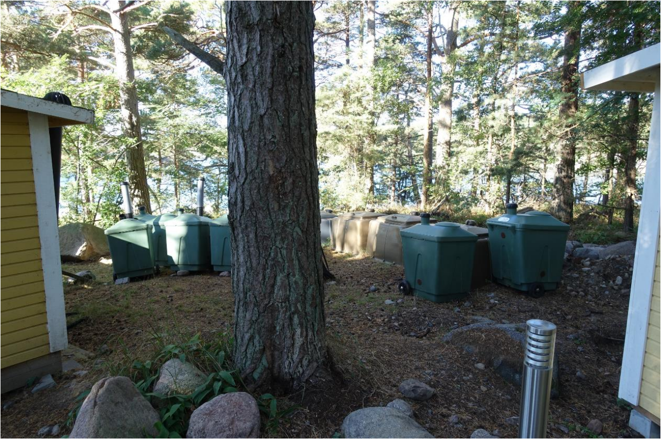
The reserve containers for the new dry toilet unit on Bodö. The lights installed in the harbour area can be seen in the photo. Photo: Metsähallitus / Sanna-Kaisa Juvonen.
