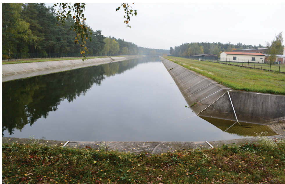
Figure 3.3 Infiltration pond in Káraný waterworks.
