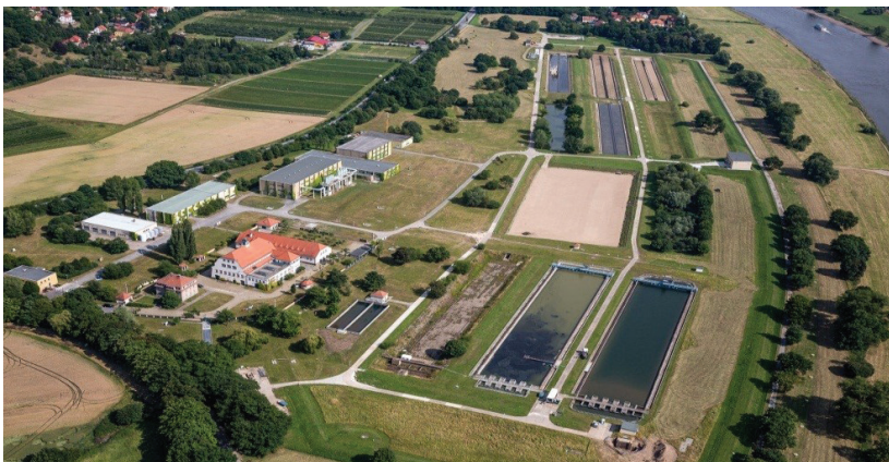
Figure 3.6 Aerial view of water works Dresden Hosterwitz (©DREWAG Netz GmbH).
