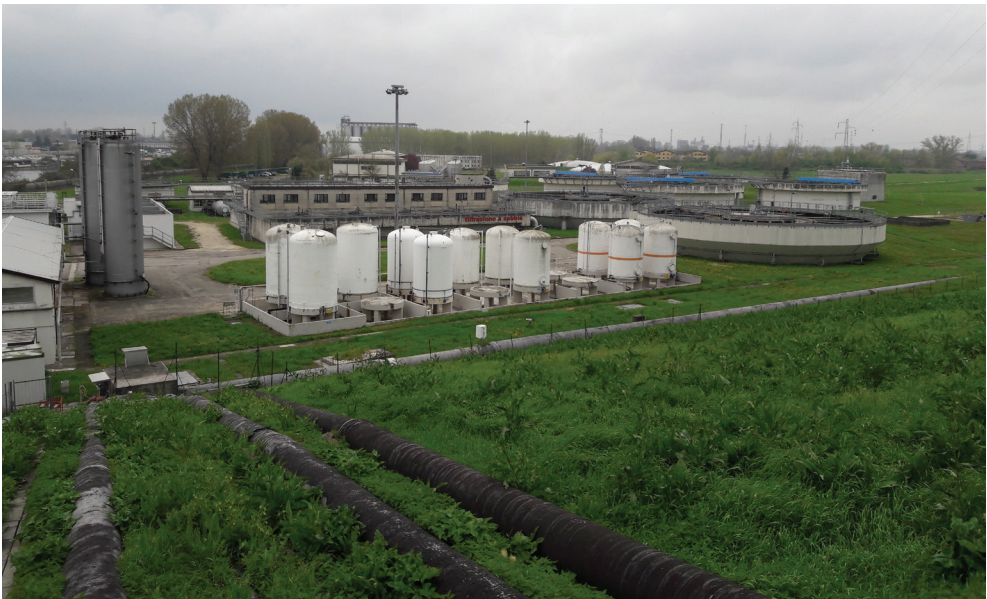
Figure 3.14 view of the Pontelagoscuro Drinking Water Treatment Plant.
