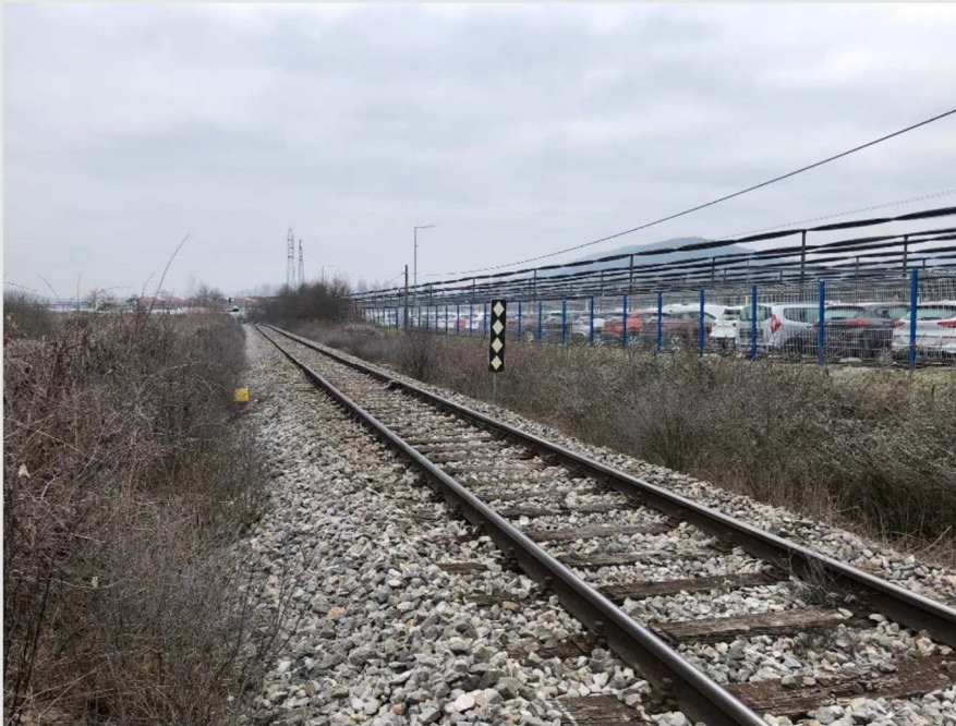
Picture 2: Location of rail switch for new siding
