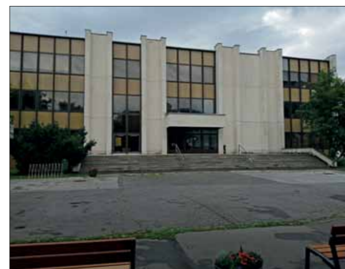
Figure 11.1 Green wall in Liptovský Mikuláš — before. Photo: P. Starek
