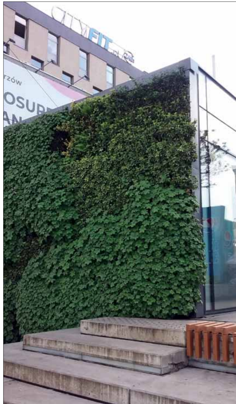
Figure 7.1.21.1 Green façade with climbing plants. Photo: J. Gorgon
