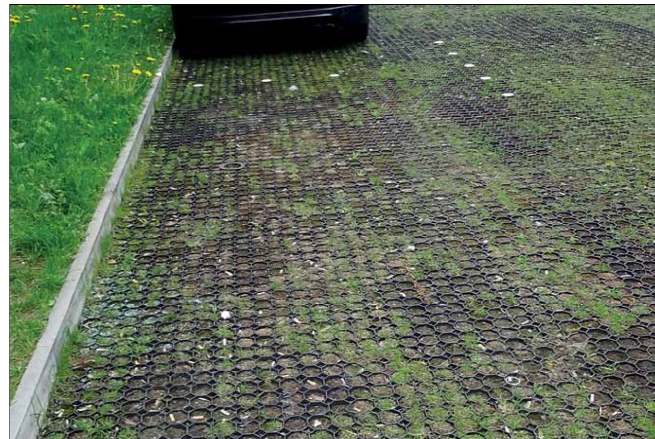
Figure 7.1.5.1 green grass pavement. Photo: B. Vojvodíková
