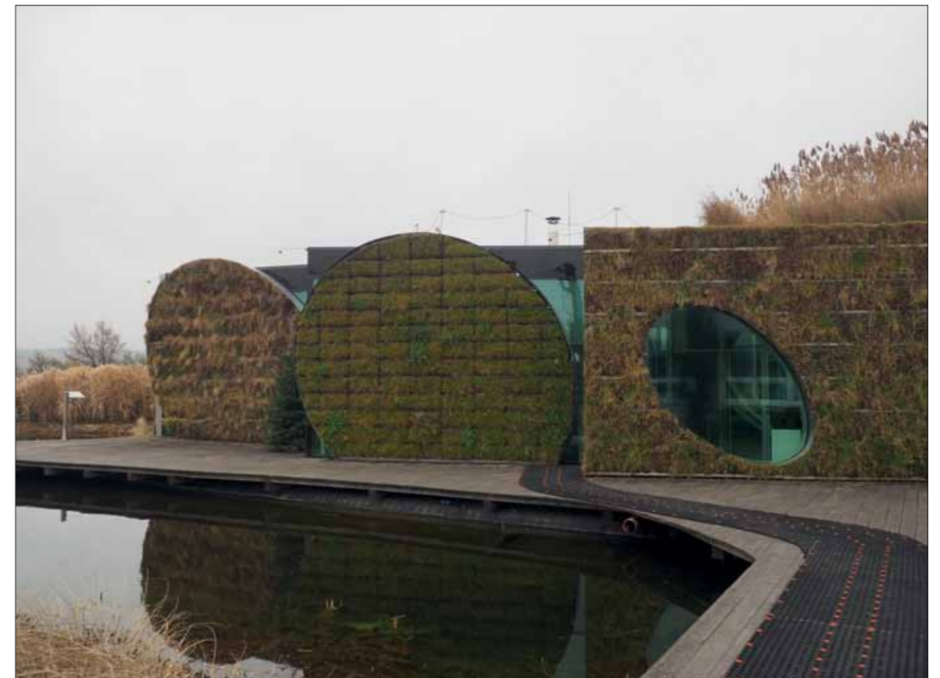
Figure 7.1.22.1 Wall-mounted living wall. Photo: A. Brázdová
