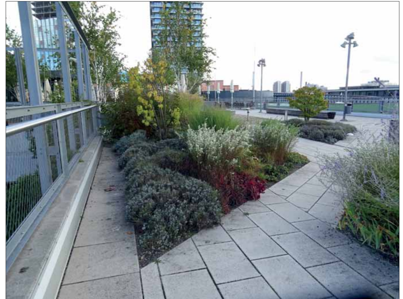
Figure 7.1.30.1 Intezive green roof. Photo: B. Vojvodíková
