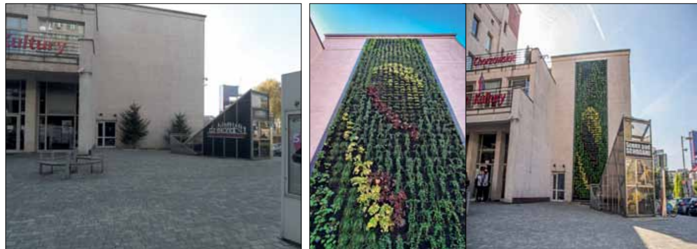
Figure 11.3 Green wall in Chorzow — before. Photo A.Beryt Figure 11.4 Green wall in Chorzow — after. Photo: A.Beryt
