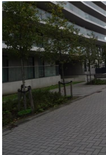
Fig. 4: A low-height swale equipped with retention layers (Photo: B. Vojvodiková)
