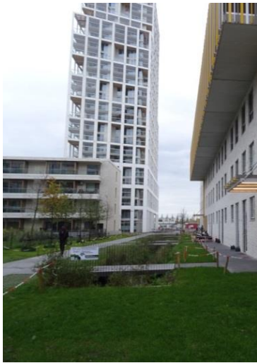
Fig. 3: Simple swales used to accumulate water from the pavement (Photo: B. Vojvodiková)
