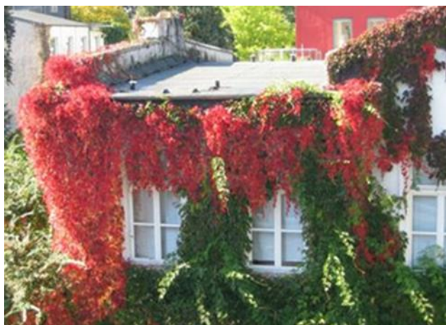
Fig. 4: Green wall (Photo: R. Bendner)
