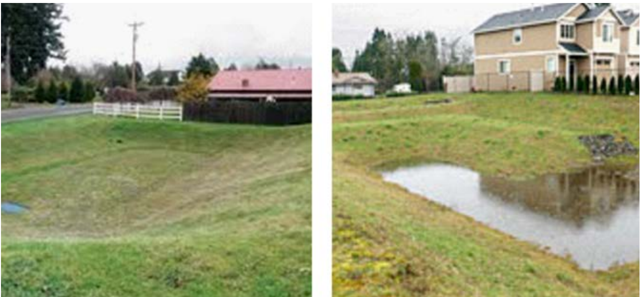
Figure 38: Empty 37 and filled infiltration basin 38 .
