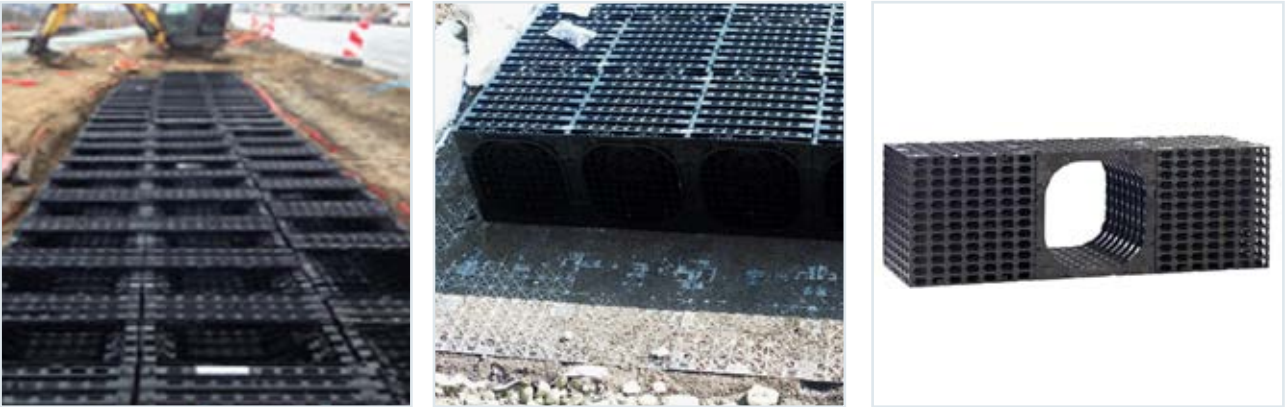
Figure 43: Trench elements (infiltration boxes) for swale-trench infiltration systems (ENREGIS).
