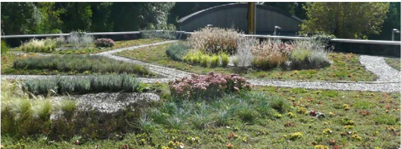
Figure 13: Intensive - perennials, grasses, shrubs - Sport facilities La Tesorina, Torino (Photo: A. Aires).
