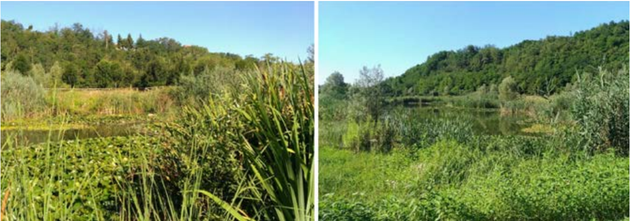
Figure 23: Examples of FWS for stormwater treatment (Source: IRIDRA Srl) 28 .
