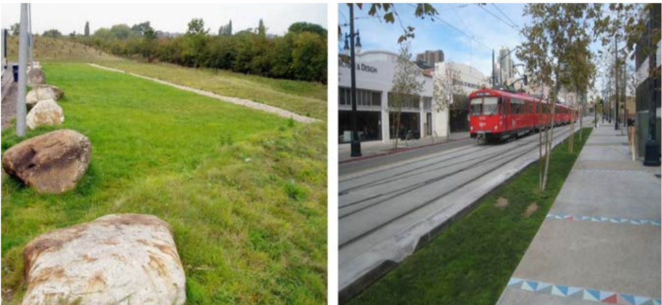
Figure 33: A filter strip adjacent to a road 36 and in the centre of town (NWRM).
