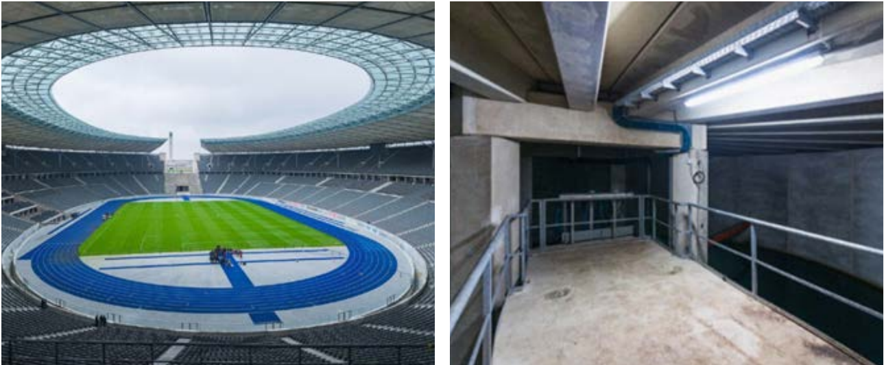
Figure 50: Berlin Olympia Stadion with stand roofing from where rainwater is collected (left) and underground rainwater cistern with different storage space levels 45 .
