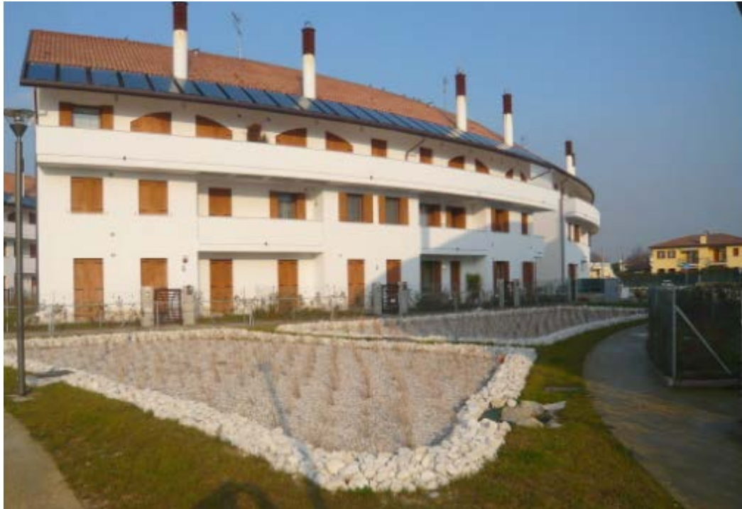
Figure 17: HF system for the separation, treatment and reuse of greywater for toilet flushing in a residential area in Preganziol (TV - Italy) 45 .
