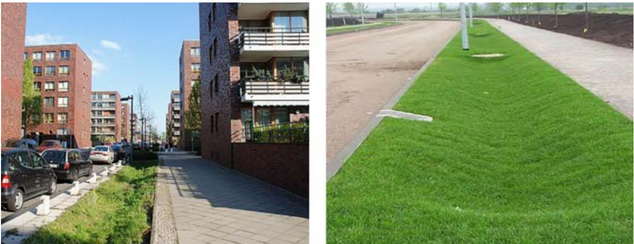
Figure 44: Swale-trench systems in Berlin (Sieker).
