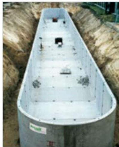
Reinforced concrete cistern (24 - 100 m 3 ) (Mall)
