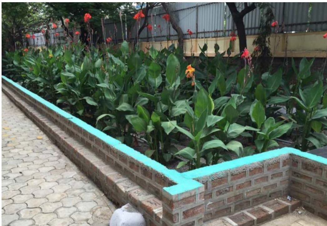
Figure 18: VF system for separation, treatment and reuse of greywater for toilet flushing in a Hostel campus of the College of Engineering, Pune (India) 45 .
