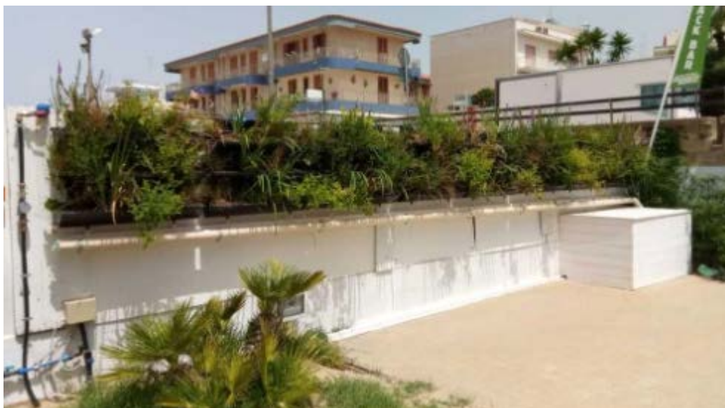
Figure 19: Green Wall for gardening reuse of treated greywater, Margarita beach, Marina di Ragusa (RG - Italy) 45 .
