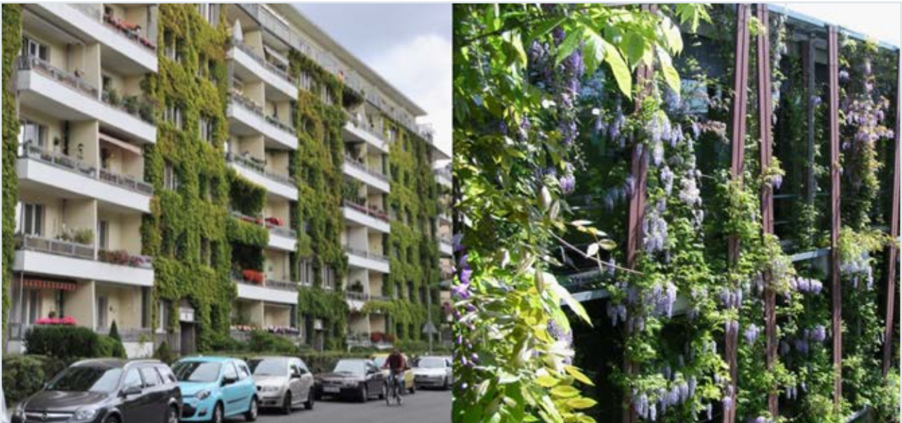
Figure 17: Ground-bound green wall with Virginia creeper (left, Photo: D. Kaiser) and system-bound green wall at the Institute of Physics in Berlin-Adlershof (Photo: M. Schmidt).
