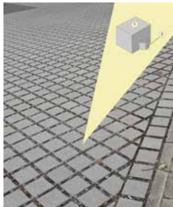
Figure 58-22: Water permeable surface of a car park: Paving with widened joints (ca. 3 cm) and principal sketch of a stone (1) with a small bulge (2) serving as spacer
