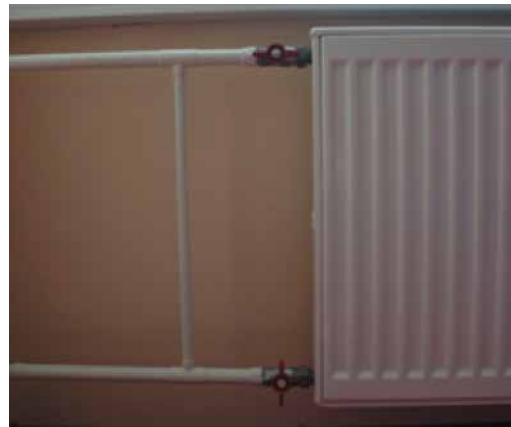
Figure 49-6: Panel radiator connection to existing single pipe system with bypass and shut-off valve
