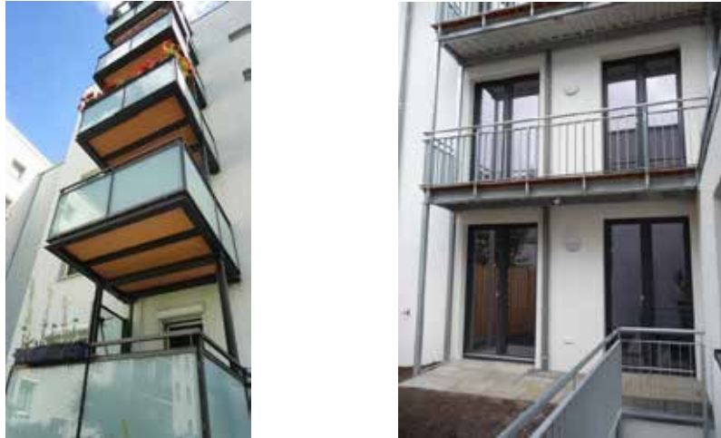
Figure 10-5: Balconies with own load-bearing structure, separate from building envelope
