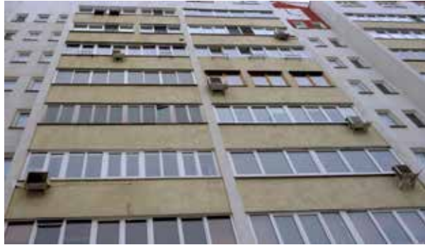
Figure 39-13: Boxes of air conditioners on facades of residential buildings can be a first indicator that overheating in summertime is an issue.
