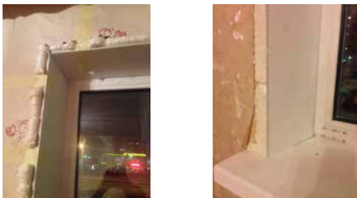
Figure 43-6: Installation foam (left), vapour seal (right)
