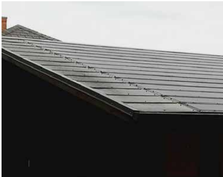
Figure 5-2: Roof-integrated system: the solar panels are almost indistinguishable from other roofing elements
