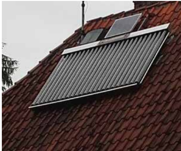
Figure 5-4: Vacuum or tube collector on the roof of a detached house
