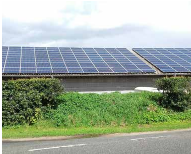
Figure 5-1: Polycrystalline modules on an agricultural building
