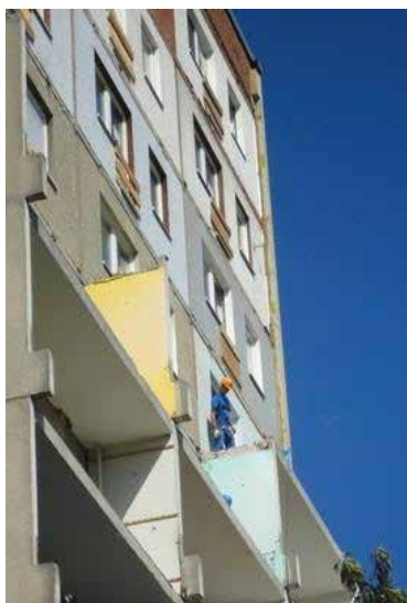
Figure 39-11: Deconstruction of balconies
