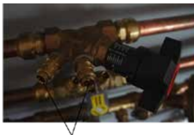
Connections for pressure drop measurements
