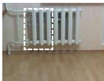
Figure 41-10: Effect of installation of heat-reflective screen. Upper left: Thermogram without screen, upper right: Heater without screen, down left; Thermogram with screen, down right: Heater with screen (marked area)
