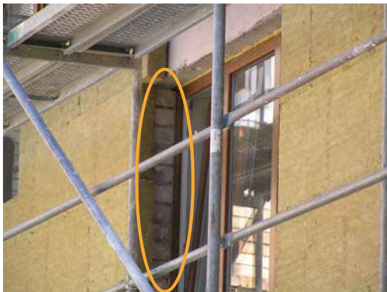
Figure 39-9: The yellow ellipse shows a potential thermal bridge. Further insulation is required to eliminate it.
