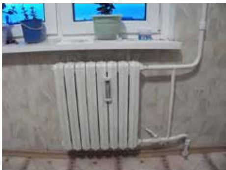
Figure 41-9: Heat cost allocator installed on heating device
