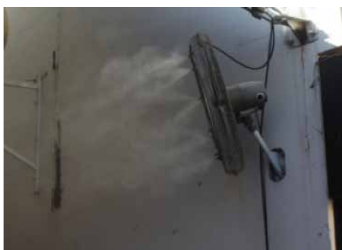
Figure 53-5: Examples of direct evaporative cooling in a restaurant in Istanbul
