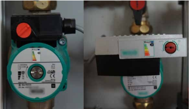
Figure 51-3: Example of circulation pumps with different efficiency classes.
