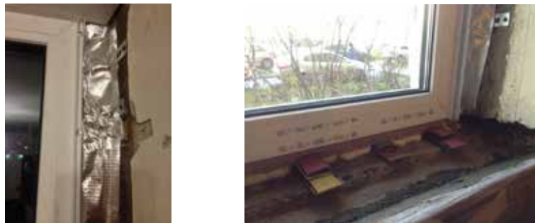
Figure 43-4: Vapour seal tape (foiled tape, left) and installation wedges, fixed with foam (right)
