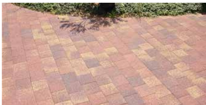
Figure 58-20: Concrete blocks with open pores structure
