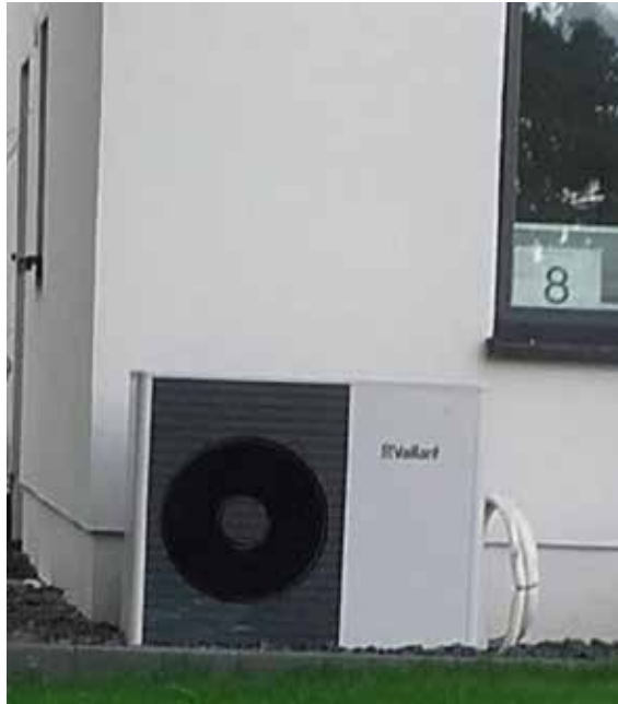
Figure 5-5: Outside unit of a heat pump
