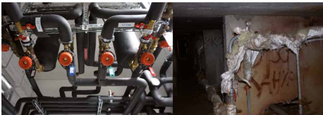
Figure 51-1: Insulated pipes and non-insulated pipes
