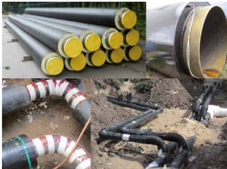
Figure 49-1: Modern pre-insulated pipes for district heating systems
