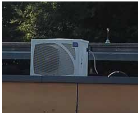
Figure 54-2: Outdoor unit of a single room air conditioner
