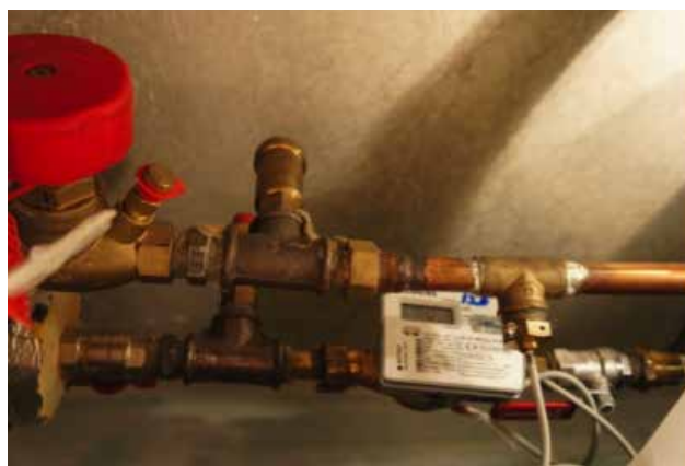
Figure 51-12: Practical installation of direct heat meter
