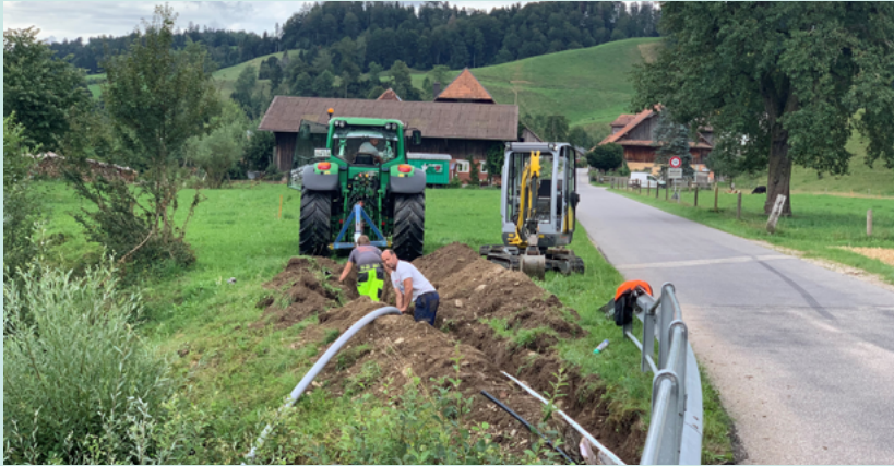
Figure 8 - The local fibre optic network of Luthern being installed (RLW)
