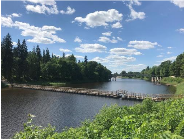
Figure 60 Example of a pontoon footbridge, Latvia (Ogre city): http://www.ogresnovads.lv/lat/pasvaldiba/projekti/zinas__jaunumi/?page=0&doc=33797
