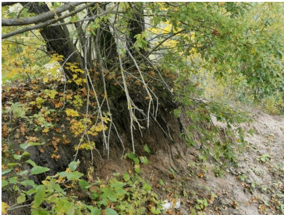
Figure 27 Sand material collapses Venta's left bank, Black Kolka (Photo I. Gavena, 2019)
