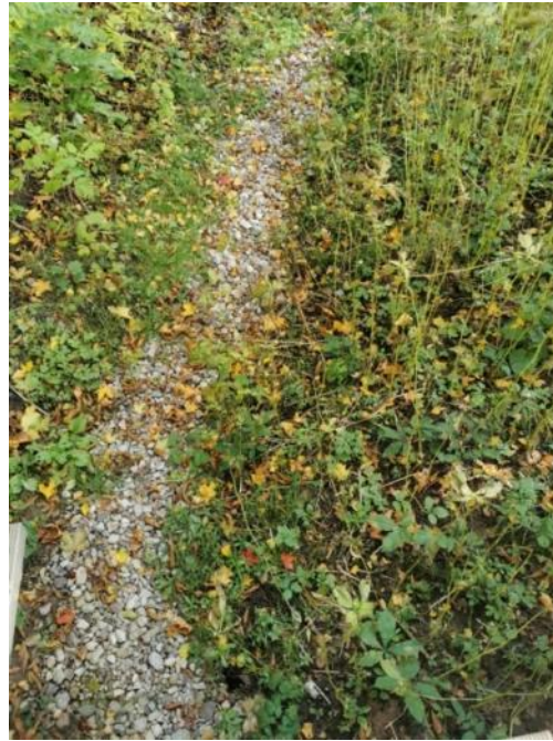
Figure 29 A ravine, the base of which is protected from deepening by the burial of pebbles – rubble, on the right bank of the Venta in the section between Ventas Street and Vidus Street (photo I. Gavēna, 2019)
