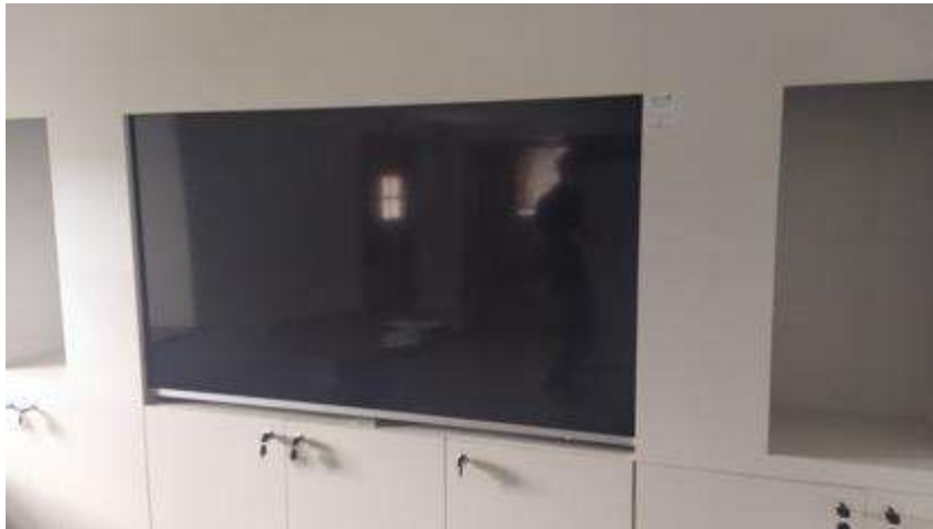
Figure 36 - Wall monitor 65", tower
