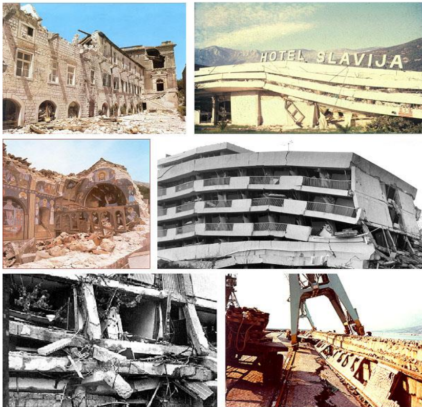
Figure 16: Illustration of the levels and types of destruction of buildings in the earthquake of April 15, 1979: detail from the old town of Budva, hotel "Slavija" in Budva, Monastery "Gradiste" in Buljarica, Hotel "Agava" in Bar, then the detail of damage in the port of Bar
