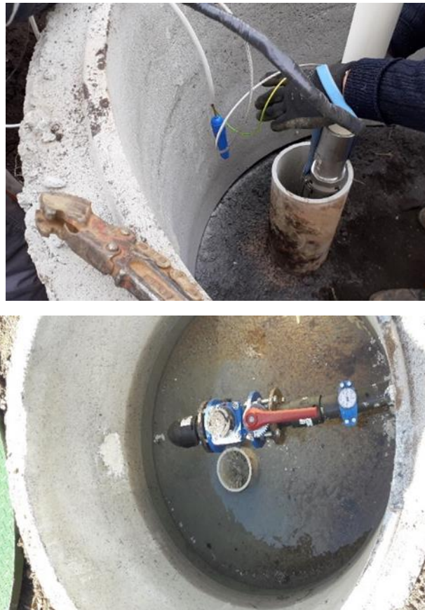
Figure 11. Grouting works and sensors' installation in extraction (up) and re-injection boreholes (down)
