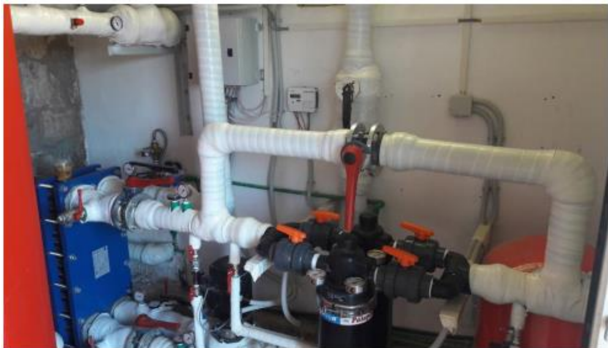
Figure 13. Heat exchanger, filters and circulation pump (primary loop)
