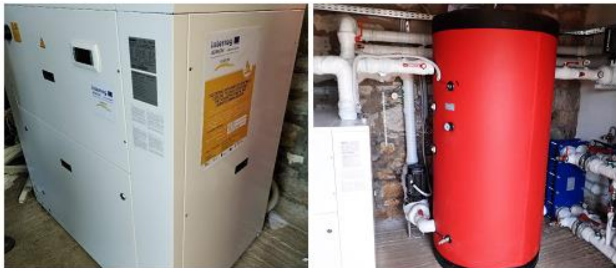
Figure 12. Geothermal Heat pump - water storage tank – heat exchanger
