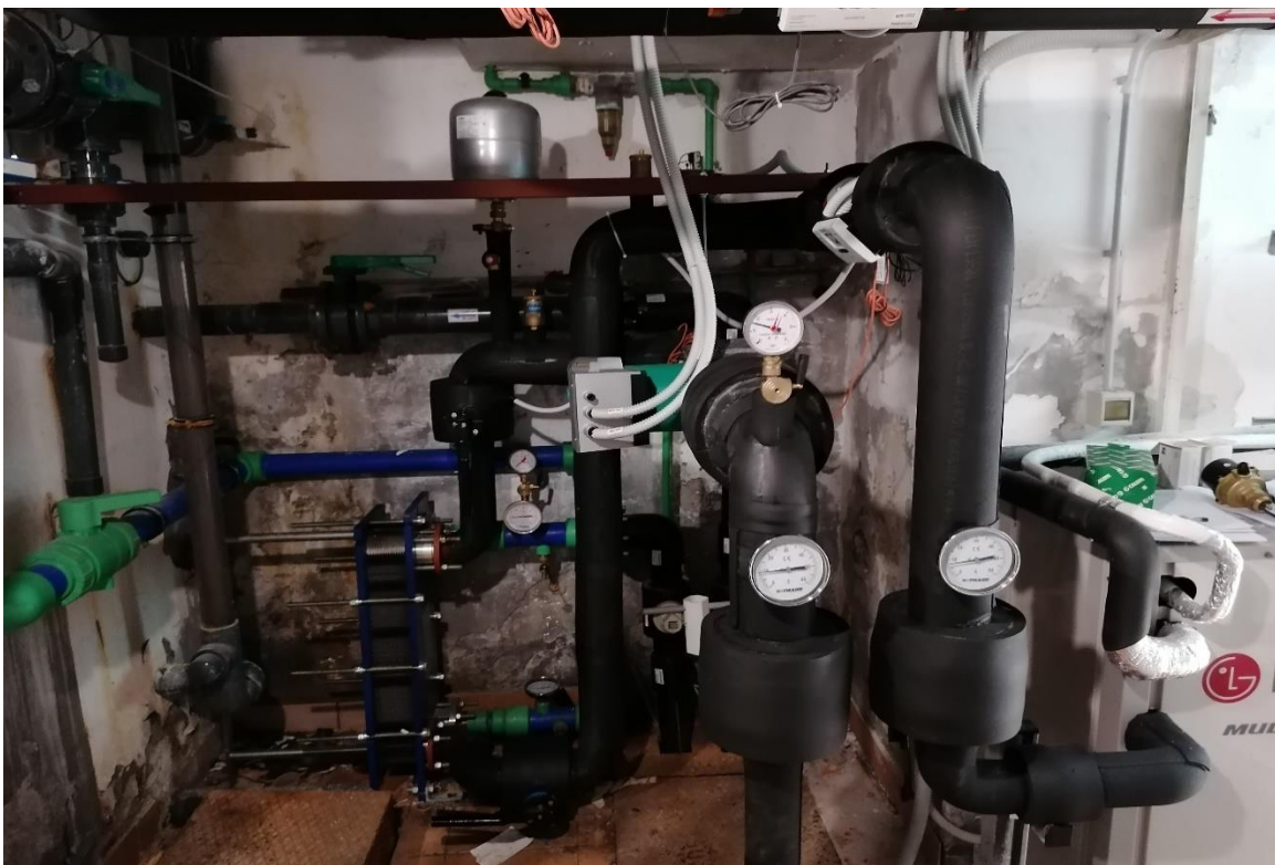
Figure 8. Heat exchanger with equipment
