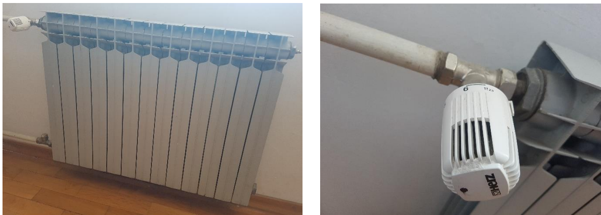
Figure 5 Heating elements (left) and built-in thermostatic valves (right) (December 2018)
