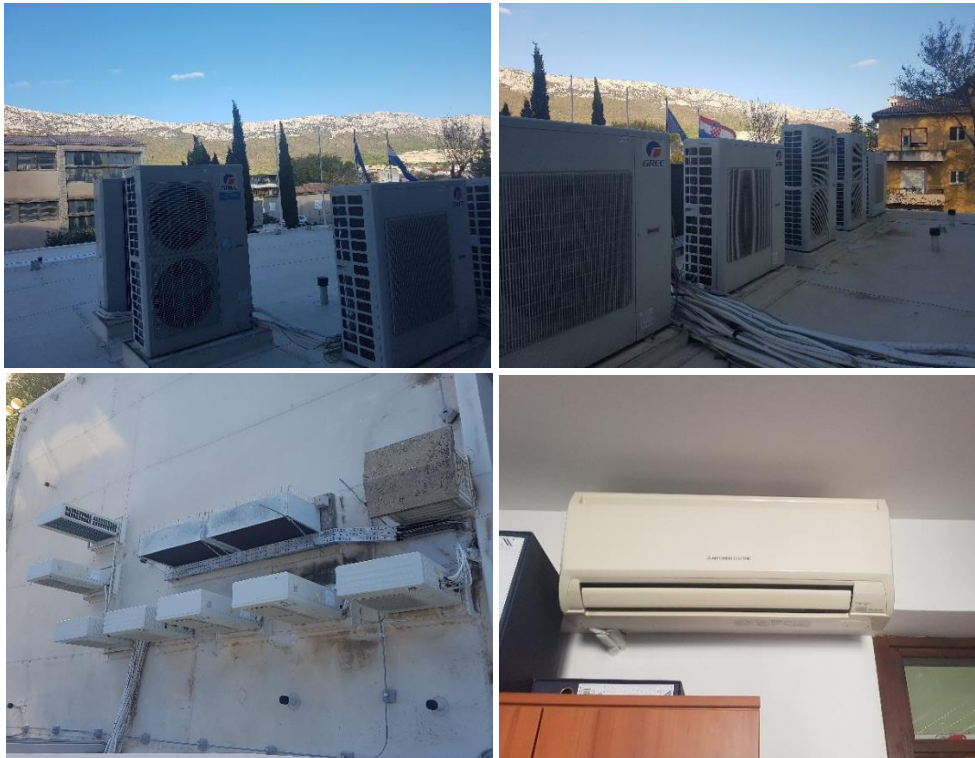
Figure 6 VRV cooling system in the city administration building in Kaštel Sućurac (December 2018)
