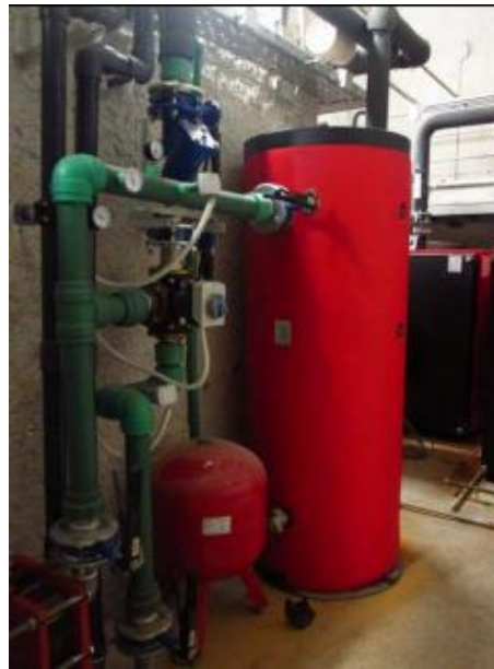
Figure 4: Heat pump and buffer tank for hot water
