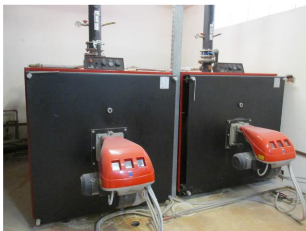
Figure 3: Boiler room for air heating
