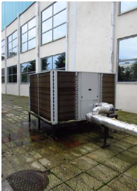
Figure 4: Heat pump and buffer tank for hot water
