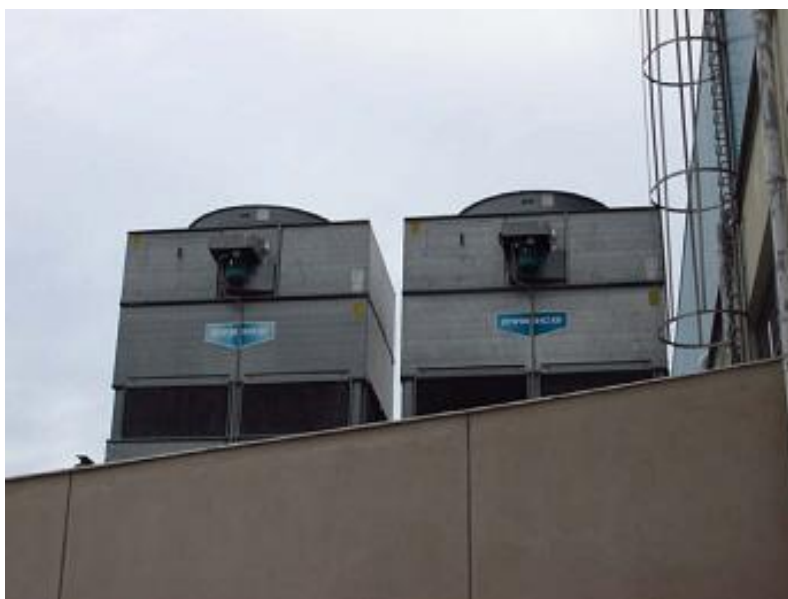
Figure 7: Cooling towers
