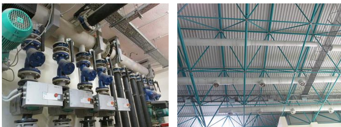
Figure 9: Piping network of AHU and Network vents on the roof of the pool
