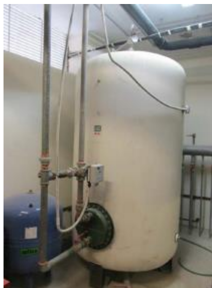
Figure 8: Boiler room for DHW production, 2000 litres
