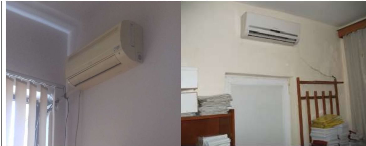
Picture 21: Using of Fan-Coil units
