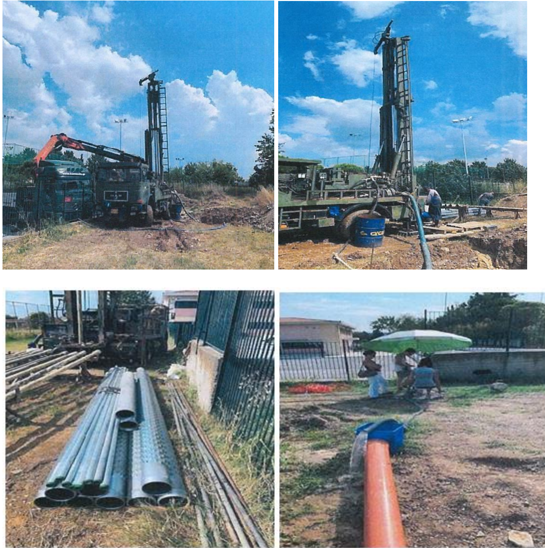
Image 3: Photos during construction
