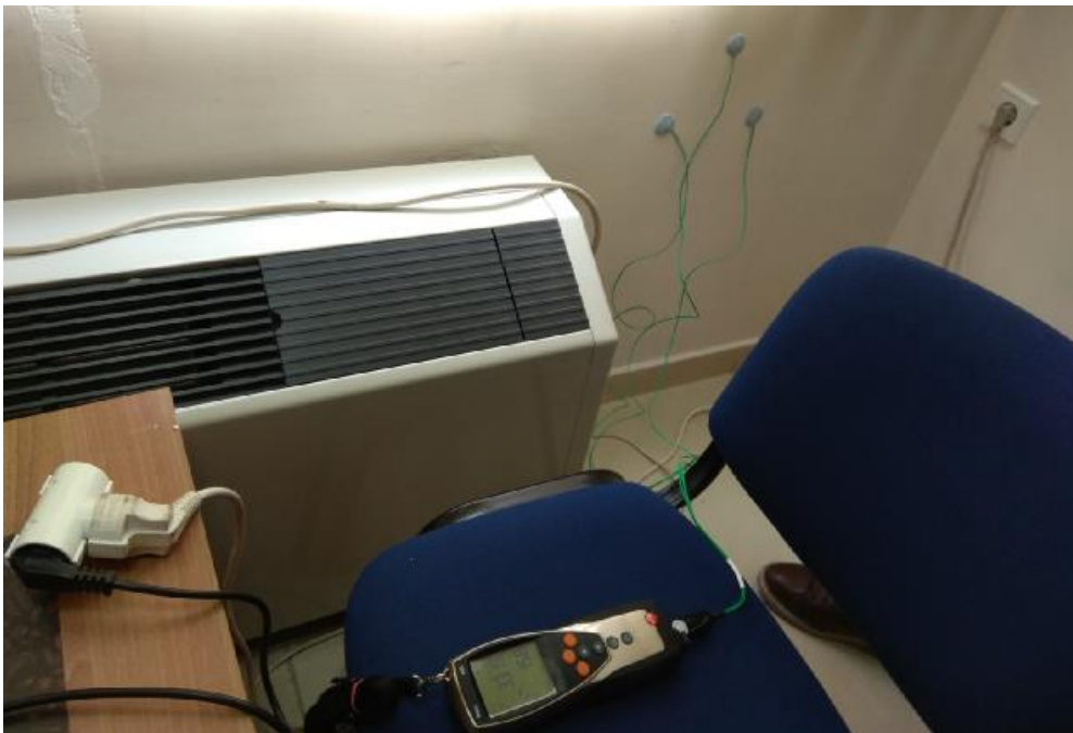
Figure 36. Measurement of heat transfer properties of an outside wall – 3 rd floor of Building B
