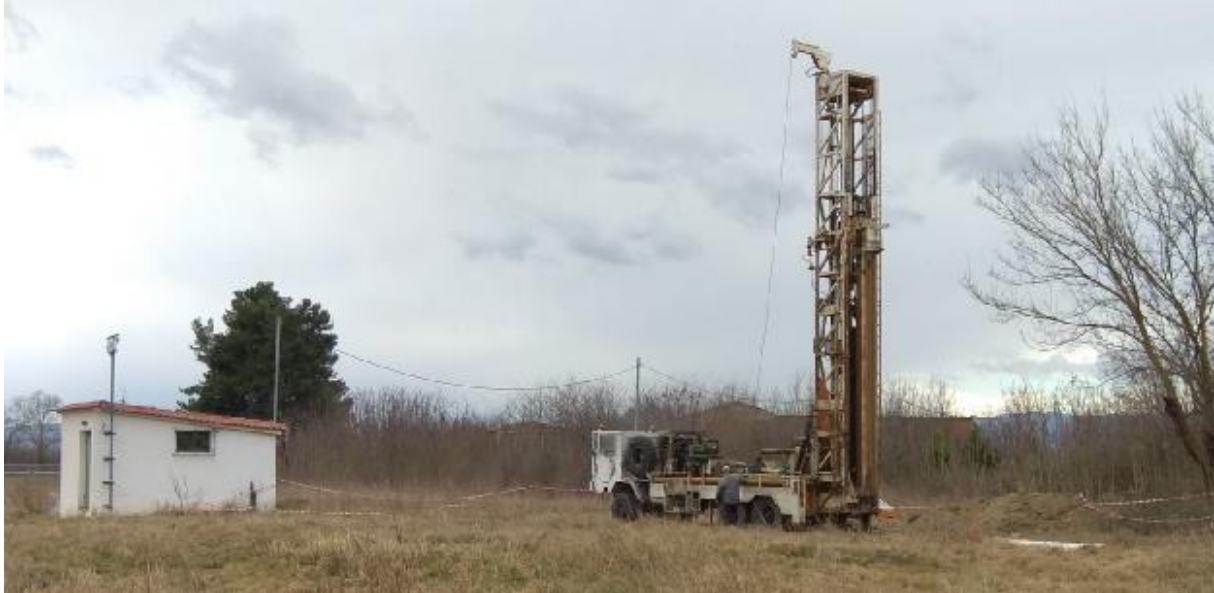
Figure 22. Installation of the drilling rig next to the excavation
