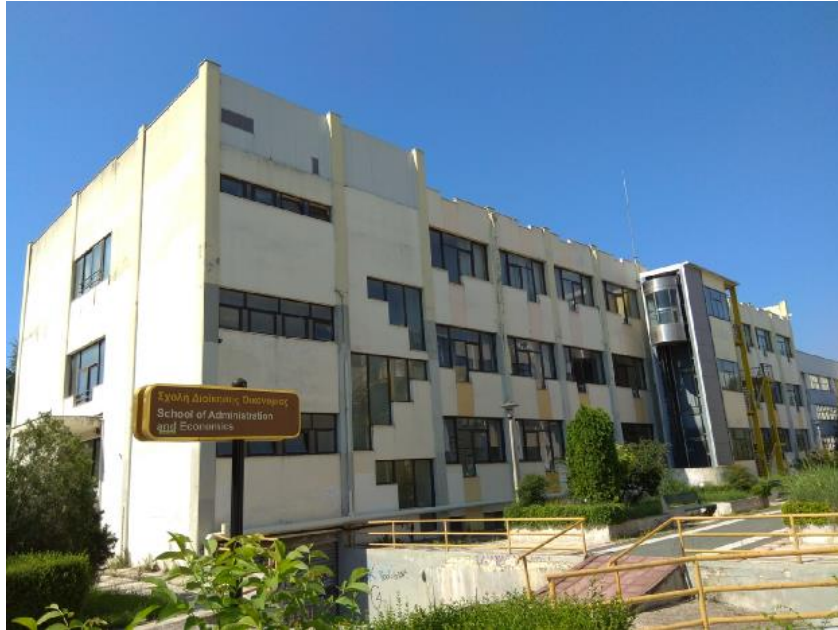
Figure 9. Front and north side view of selected Building B for the studies.
